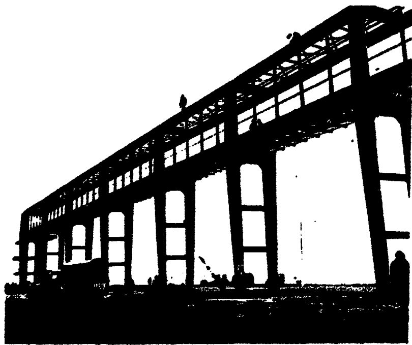
Bulk handling installations of the new port of Eilat
