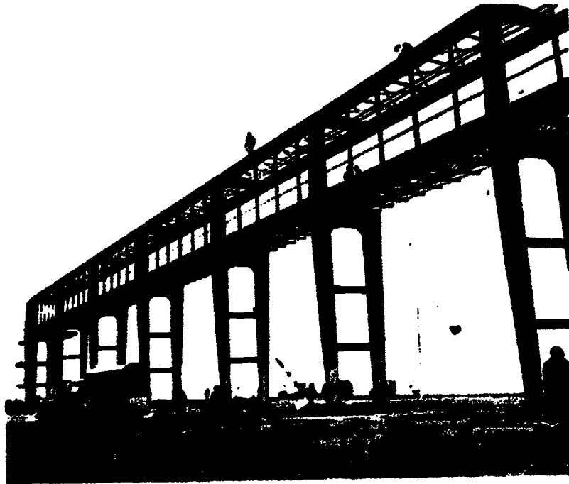
Bulk handling installations of the new port of Eilat
