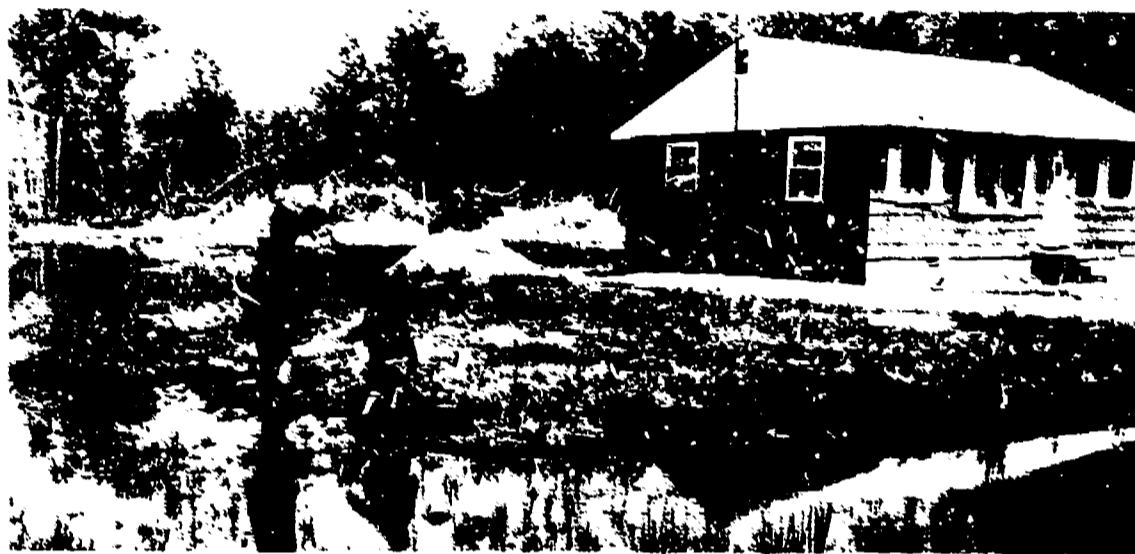
This site appeared desirable when home was built during dry season. Soil survey would have indicated extreme wetness after heavy rains or spring thaw.
