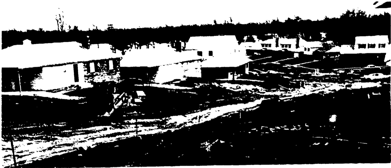
Construction of new homes near Largo, Md., a suburb of Washington.
