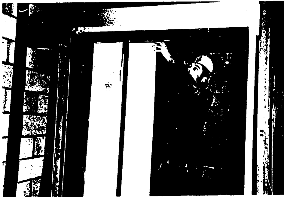
Elevator constructor adjusts door.
