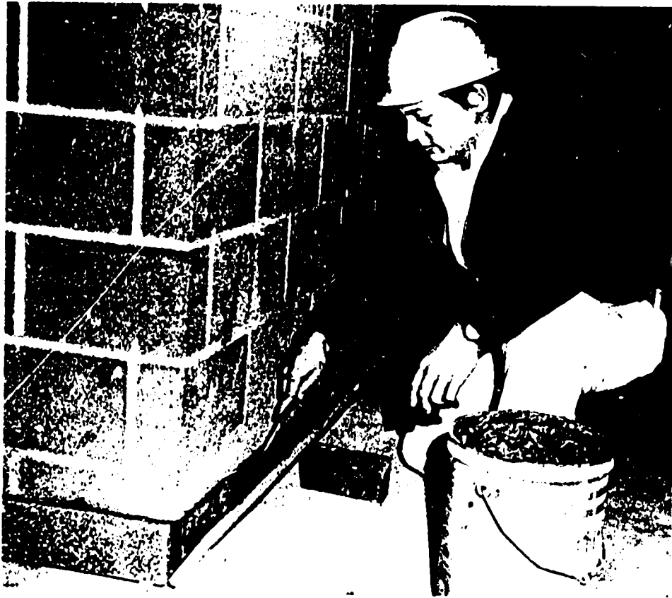
Marble setter applies mortar to terrazzo panel.
