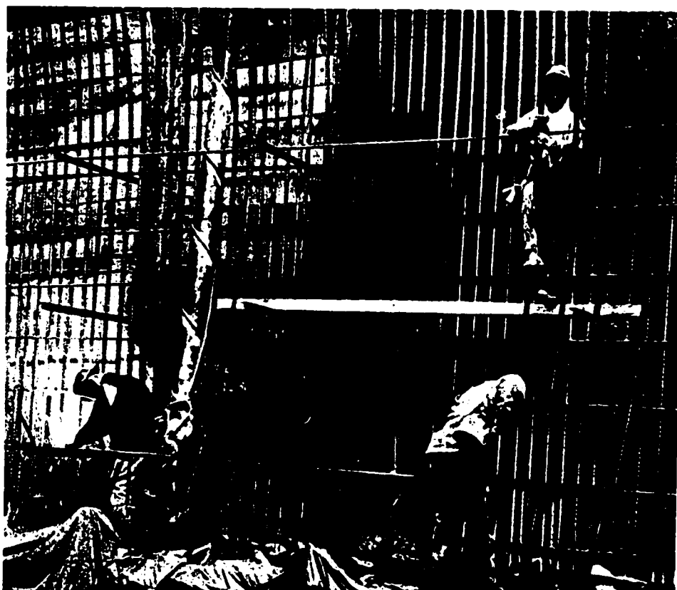
Rodmen position reinforcing bars.
