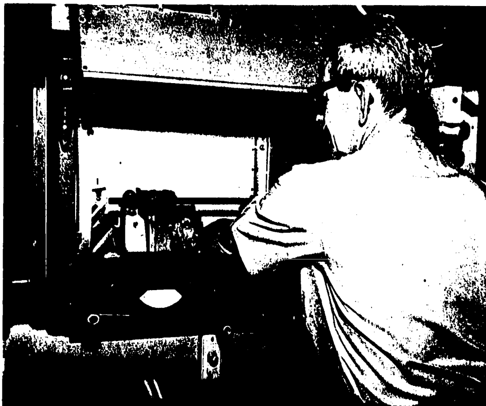
Projectionist adjusts carbon arc lamp in projector.
