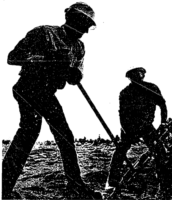
Line construction crewmen tighten a cable supporting a guide mast tower for the Pacific Northwest-Southwest Intertie.
