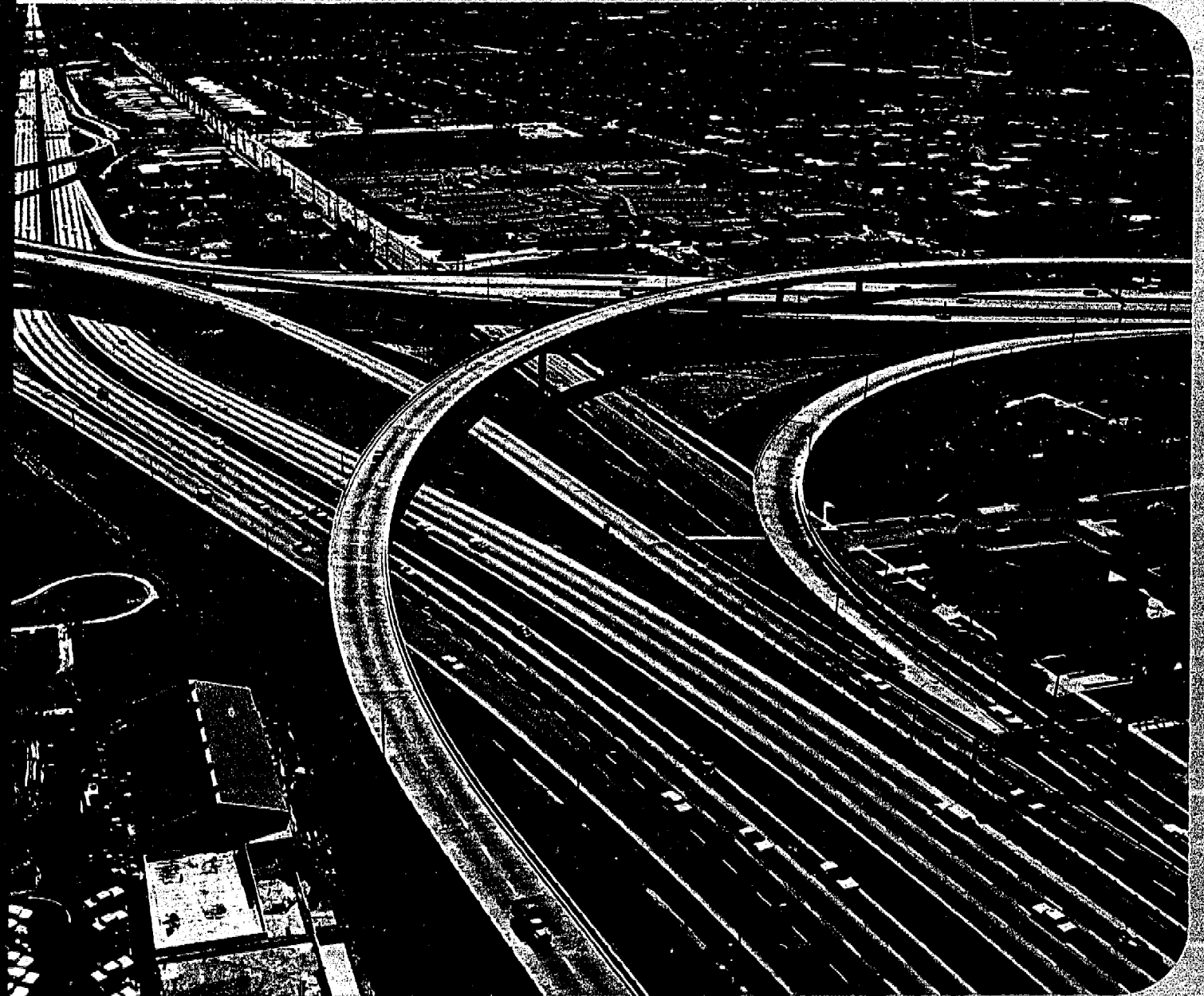
Aerial shots of super highways illustrate dramatically the amount of green open space which has "gone under" in the cause of speed and motion.
