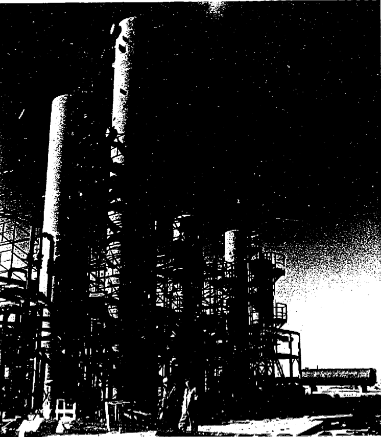
The freezing process for converting sea water to fresh is near readiness at Wrightsville Beach, N. C.
