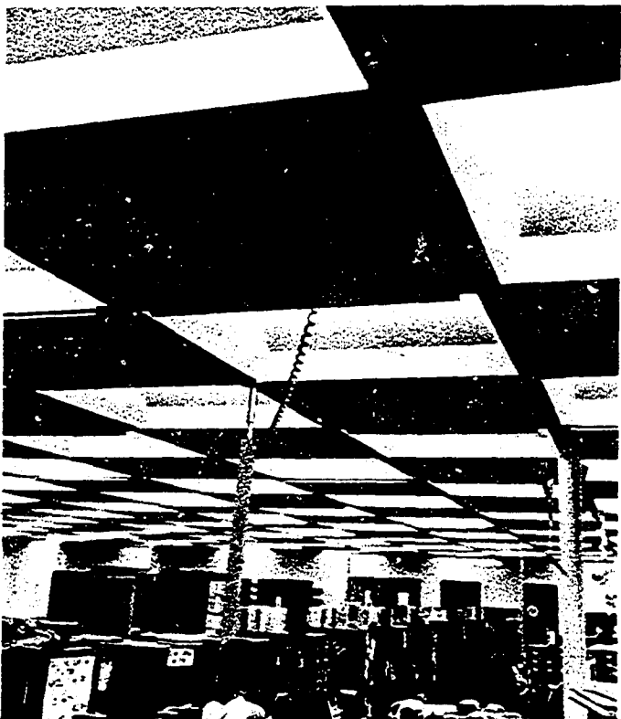
Even in schools without sophisticated distribution systems, band-aid devices can be installed. After this open school was completed, there was a need for additional local power sources. Movable pogo sticks solved problem by tapping into ceiling power.
