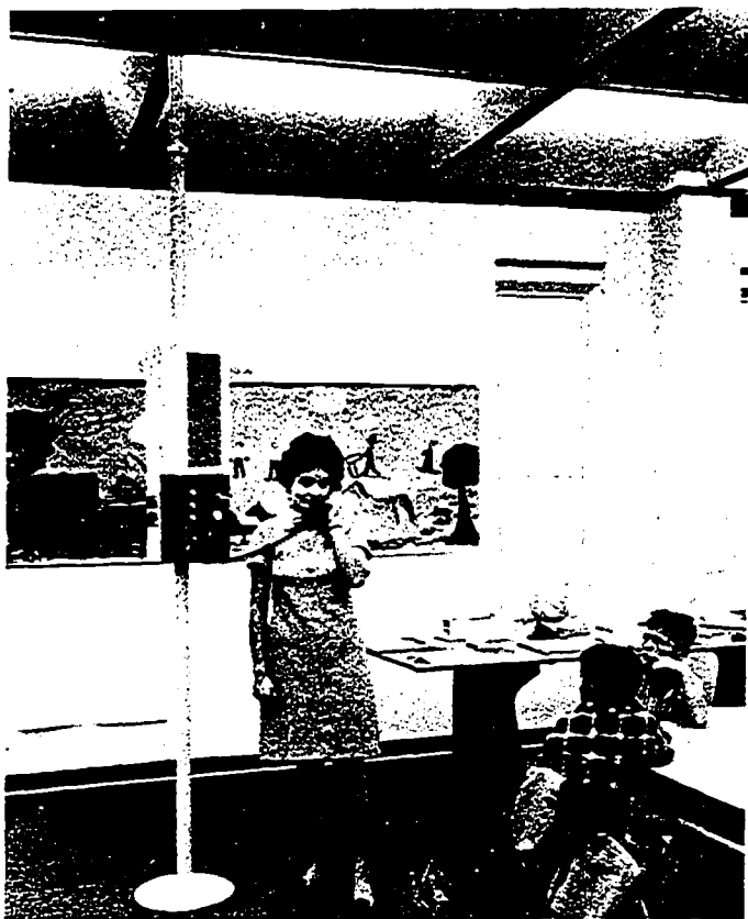
Ceiling power. Down-delivery system, designed here as an integral sub-system of the total structure, has spring-loaded poles that tap power and communication source through ceiling. Poles can be easily relocated to provide power and communication outlets almost anywhere within the room.
