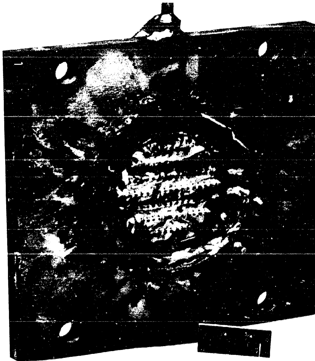
FIGURE 3-3. Erosive effects from high-frequency "screaming." Instabilities in a combustion chamber caused severe erosion of this fuel injector plate. Burnout of this plate occurred in about 0.5 sec.
