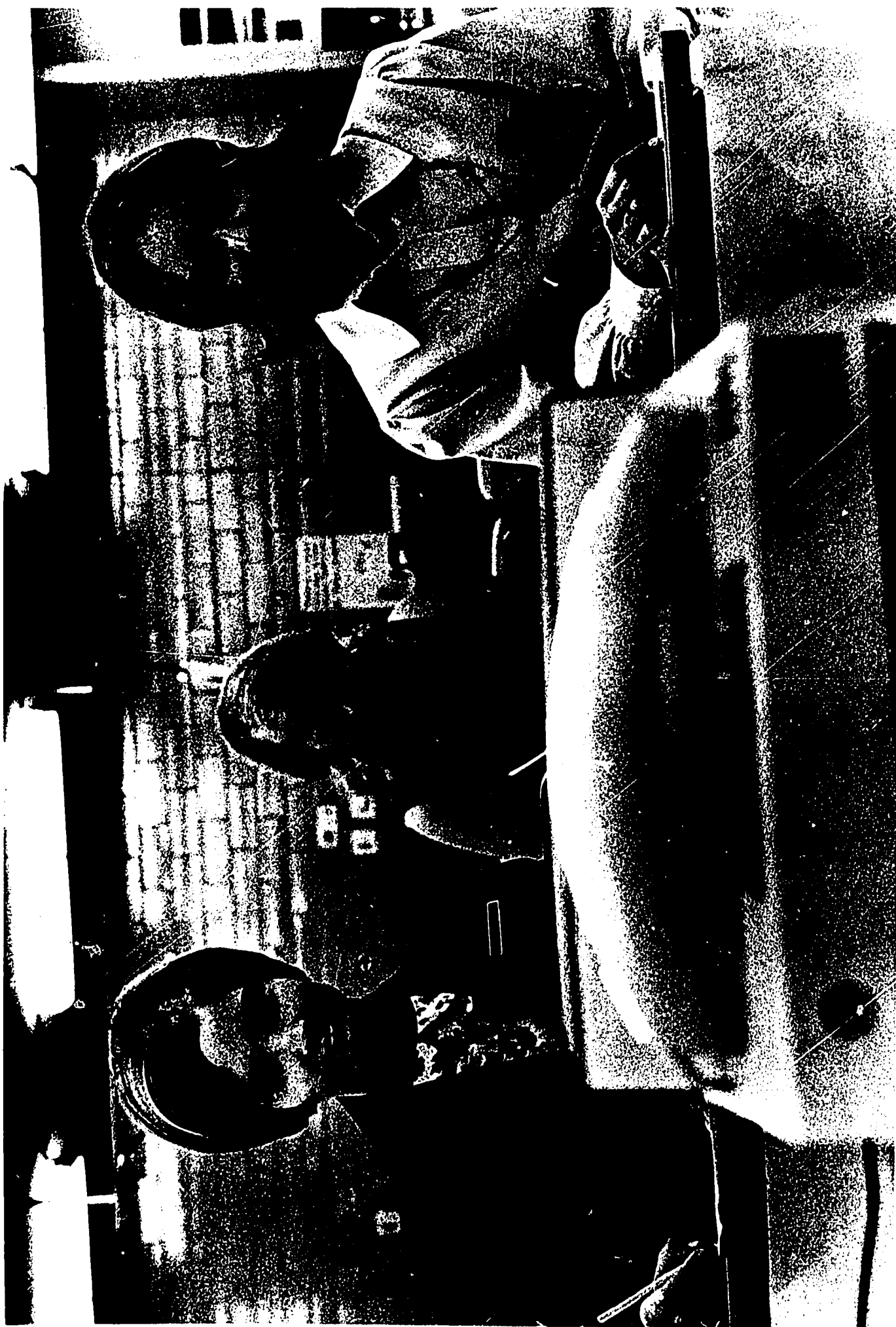
NURSES in a West Virginia hospital listen to a lecture on the growth and development of human beings. The lecture is being broadcast by the Bell System's new portable conference telephone set, foreground. The telephone, roughly the size of a shoe box, can be a "stand-in" teacher that can transmit live and taped lectures from far-away medical experts to an audience of 50 people. The set is made by Western Electric, the people who make Bell telephones and the communications equipment of the future, at the company's Shreveport (La.) Works.
