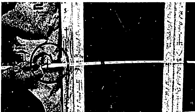
Fig. 61A-6. Measure Across for Pipe Location
