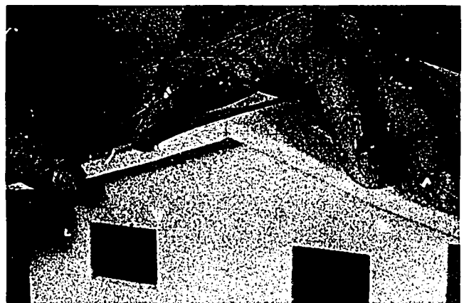
Fig. 85A-5. Checking Roof Ridge for Fit
