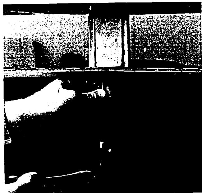
Fig. 58B-2. Setting Finish Nails in Soffit (Fascia has been removed to show how the nail set is held.)
