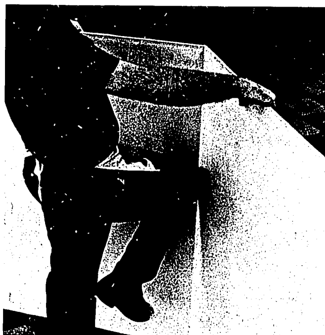
Fig. 61A-3. Applying Pressure Along Scored Line
