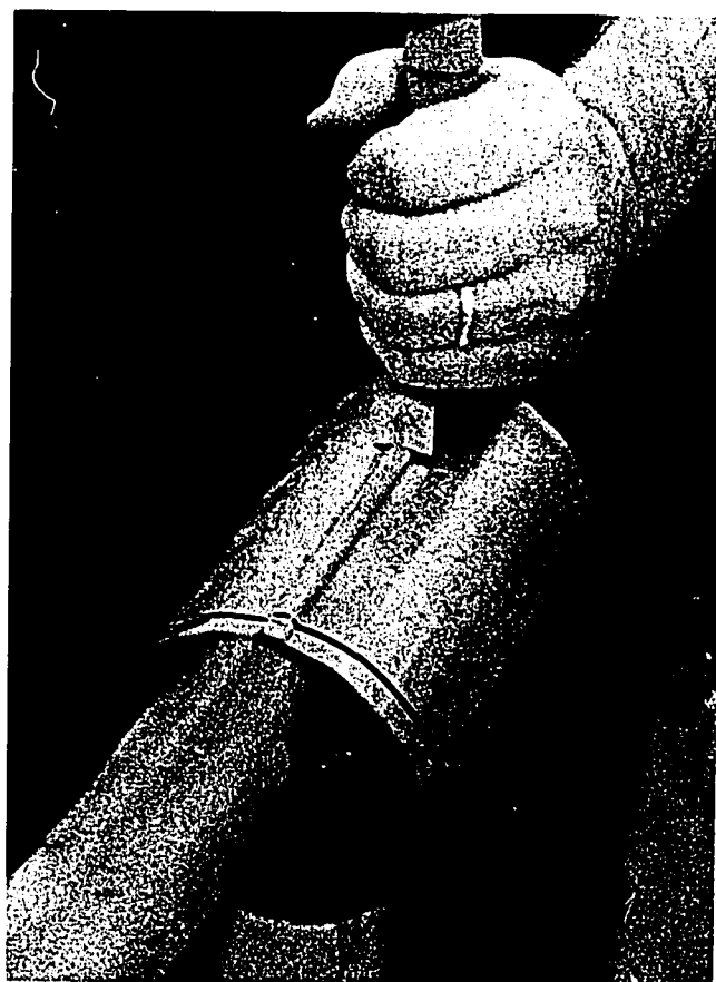
Fig. 49A-11. Finishing the Duct Seam
