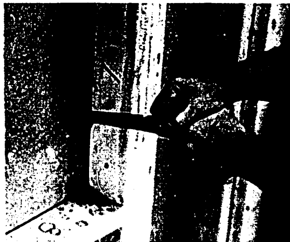
Fig. 56-5. Cutting Window Opening
