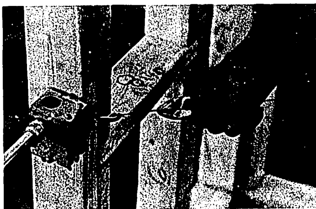
Fig. 53-10. Pulling T.W. Wires Through Conduit
