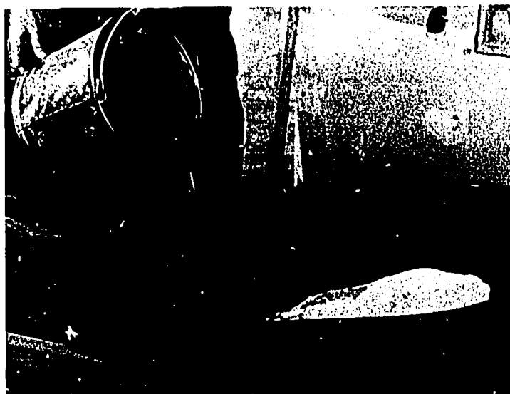
Fig. 61D-1. Water Is Poured Beside Plaster, Not on Top
