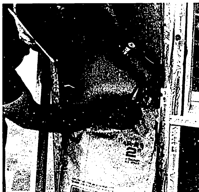
Fig. 60-6. Fitting Insulation Around Electrical Outlet
