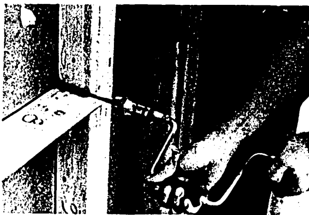
Fig. 56-4. Boring Starter Holes
