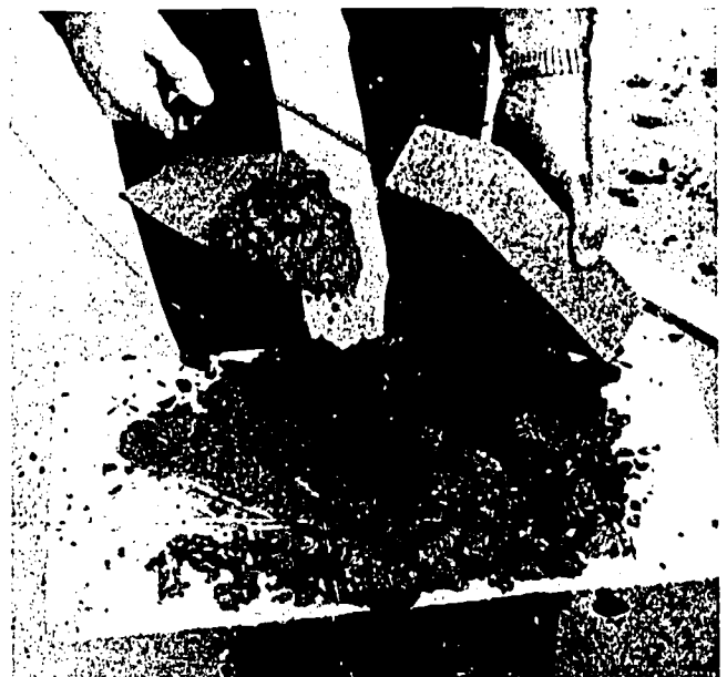
Fig. 58E-2. Mortar Ready for Buttering
