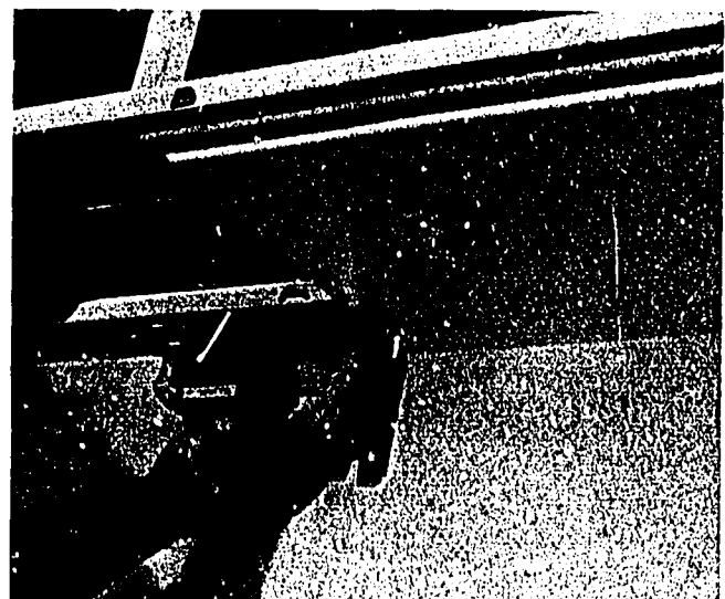
Fig. 62-4. Tile in Position for Stapling
