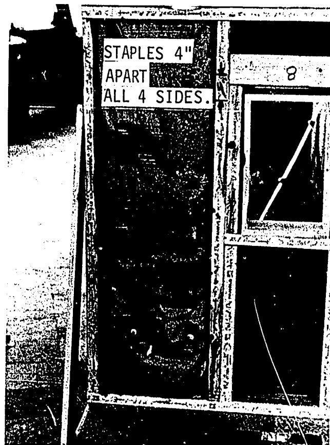
Fig. 60-8. Blanket Insulation Installed in One Section of Wall
