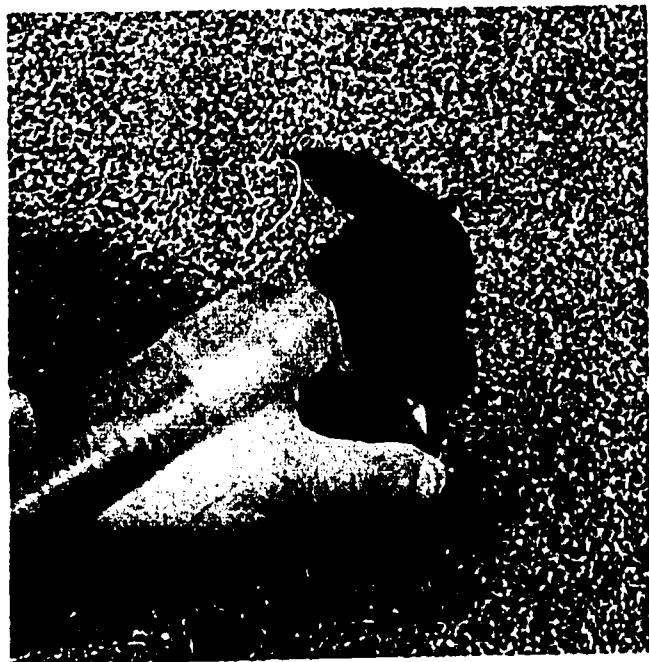
Fig. 30-2. Driving Corner Pins
