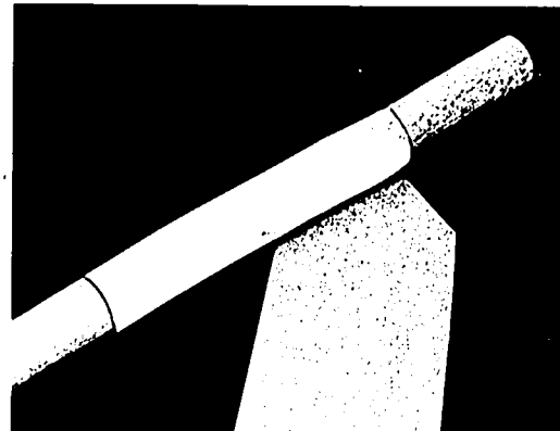
Fig. 4A-18. Positioning Angled Tape
