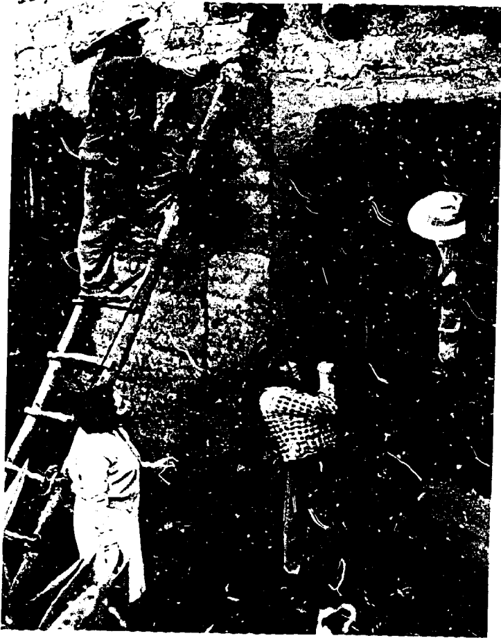
On the home improvement worker's advice, this family in Ecuador repaired the cracks in the walls of their home before they put on a new coat of plaster.
