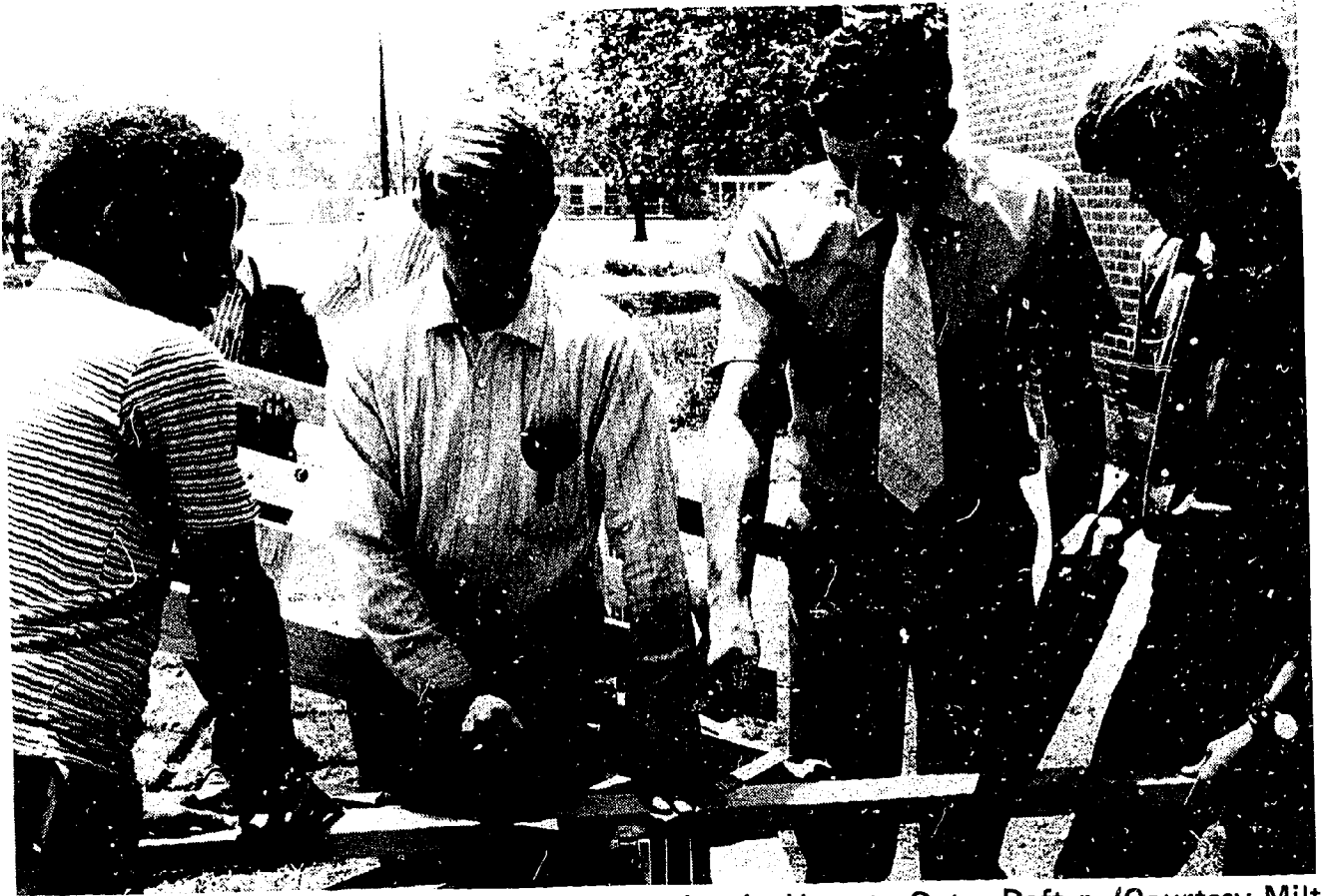
High School Students Receiving Instruction in How to Cut a Rafter. (Courtesy Milt Lawrence, Jackson, Mississippi.)
