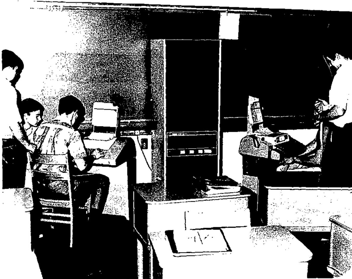
A PDP -8/I computer installed in the Salem School District. One Teletype serves as input-output for the 8/I and one is used as a remote terminal to G. E. Time-Sharing.
