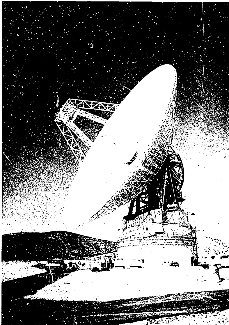
The 64 m diameter antenna of the Goldstone, California, earth station
