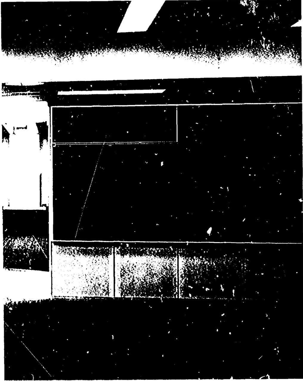
This view is from one classroom looking at and across the corridor to another classroom. As may be seen, the corridor has a hung ceiling with grills facing the classroom areas. These are intake or exhaust grills and the enclosed space above the ceiling serves as a return air plenum for proper air circulation.
