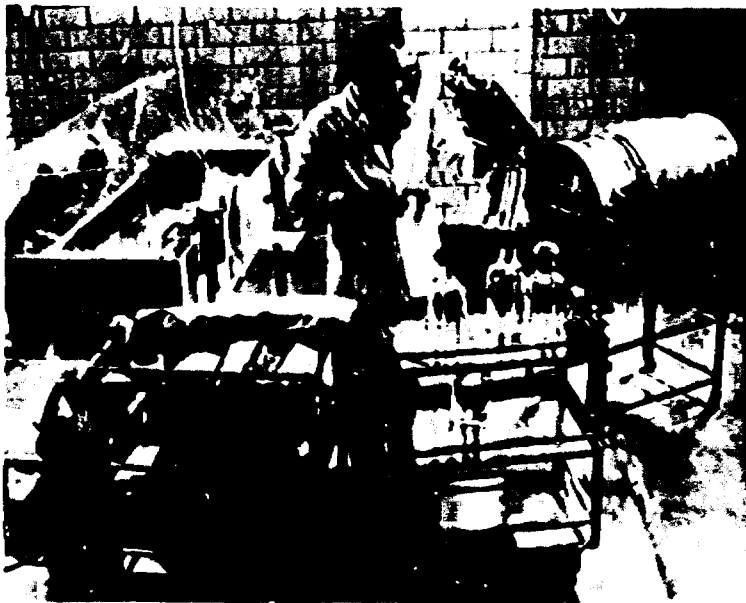
A technician sprays water bottles in one of the many steps necessary in preparing a germ-free environment for mice. On the right is a cylinder containing food and bedding and on the left is an isolator with rubber gloves for manipulating the environment from the outside. Food and water are transferred into the isolator in a careful procedure designed to keep pathogenic organisms at a minimum.
