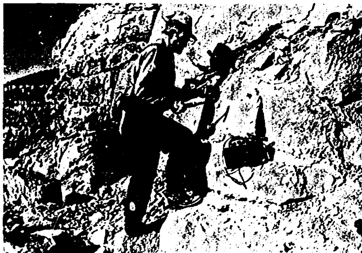
Prospecting for uranium with hammer and Geiger counter.
