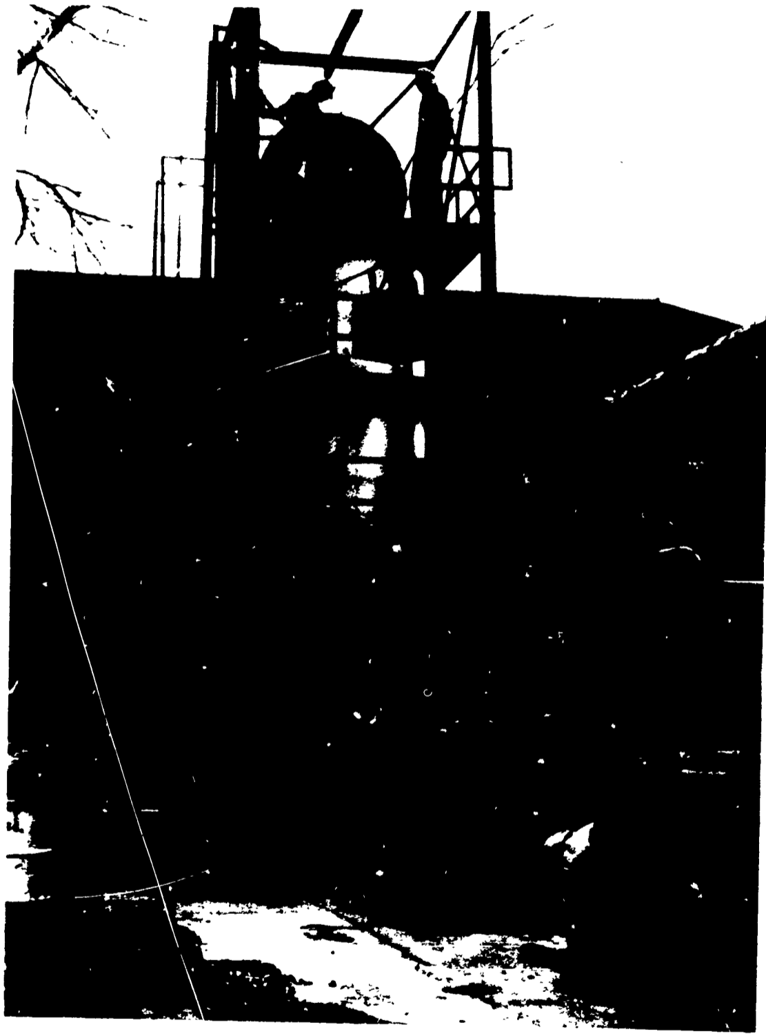
Fig. 11—Loading the 10-ton retort for the oil-shale retorting experiment.
