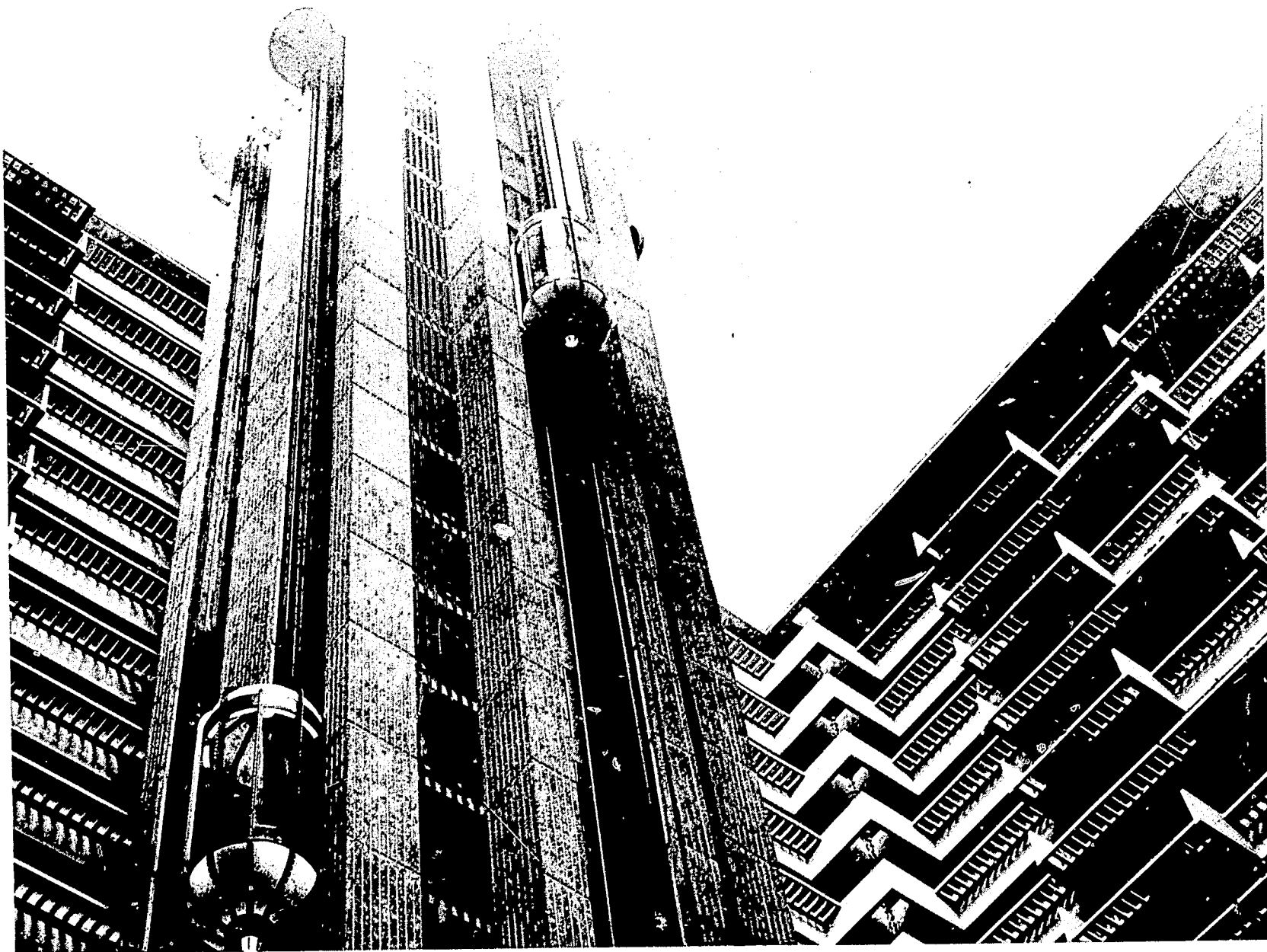
Figure 2.—This view of two of the five elevators which serve the lobby of a 30-story hotel building illustrates a type of structure on which architects, construction engineers, and technicians should work together from the beginning of the designing until it is completely built.
