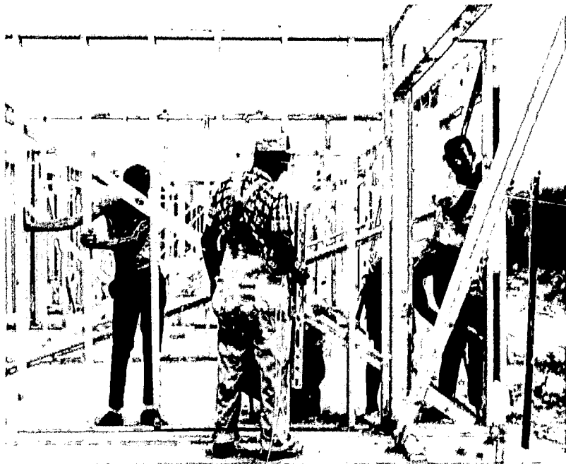
Figure 8.—Wood frame building and construction such as that shown here still represents a large and important part of the Nation's building. Technicians must understand this kind of construction.
