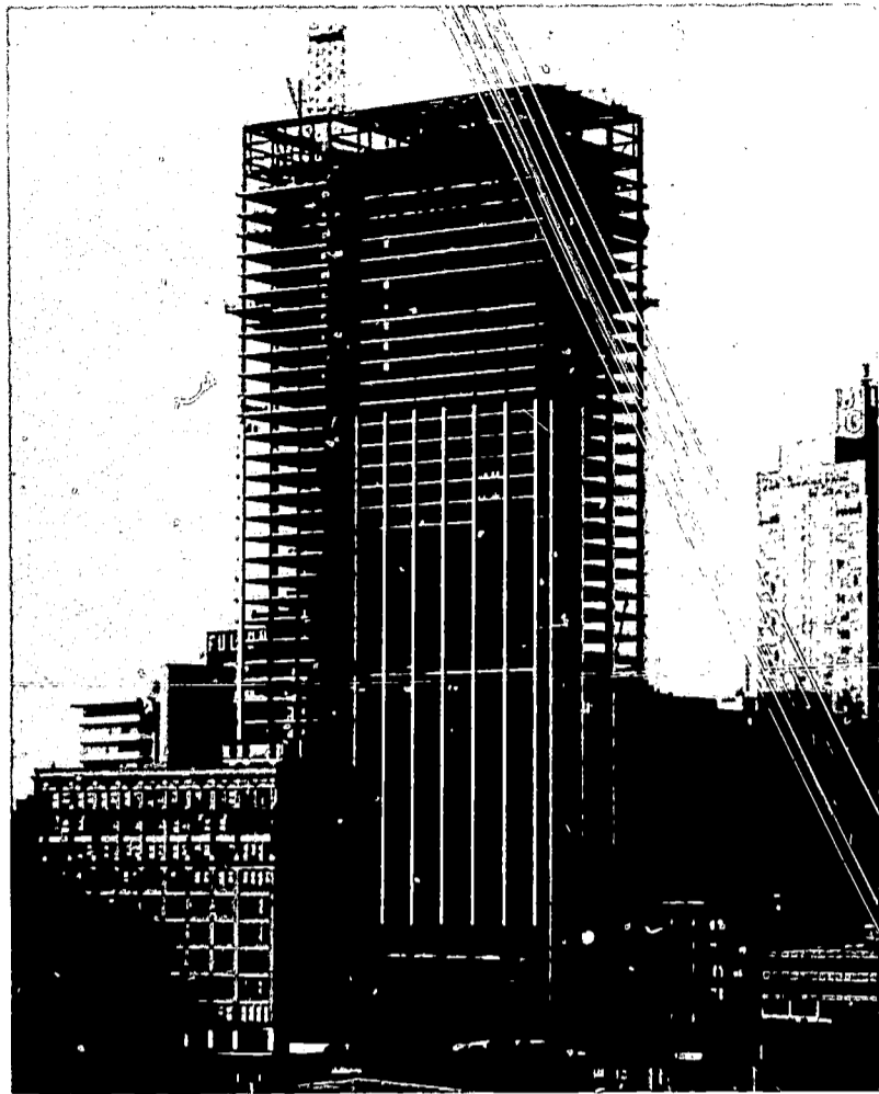
Figure 6.—Most of the elements of the structural steel frame for this building were prefabricated in factories, shipped to the building site, and erected. This includes curtain wall elements as well as steel framing. Technicians must understand the critical path method of planning and controlling such modern construction.
