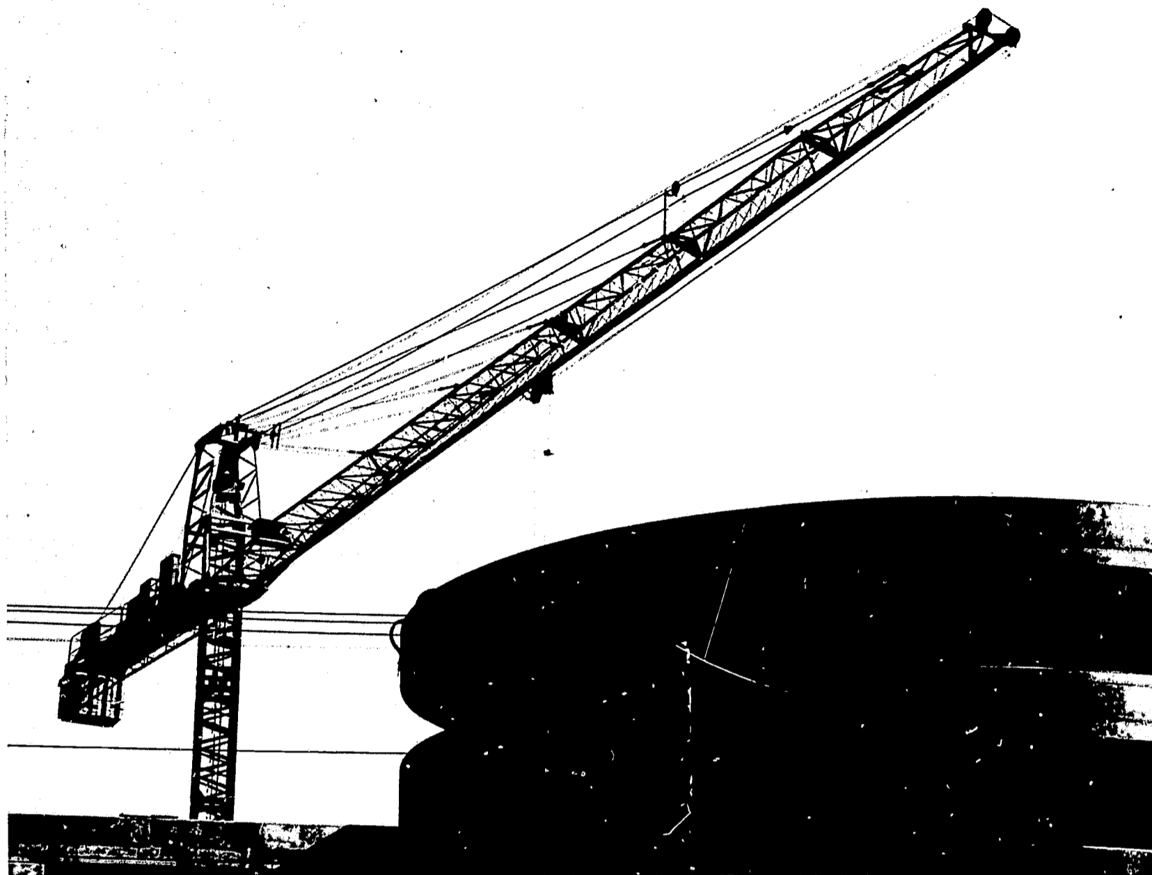
Figure 3.—New kinds of construction machinery such as this gantry crane and novel and efficient uses of materials permit freedom of architectural design until recently unknown in building construction.
