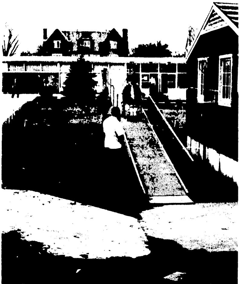
Figure 1. Ramp without rest platform.
