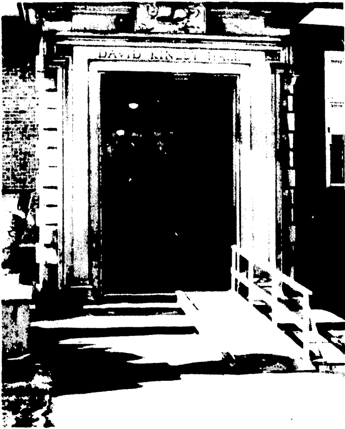
Figures 5 & 6. Much-used University building has been equipped with ramps outside and inside of entrance door, with one door shortened and re-hinged, to accommodate wheelchairs.
