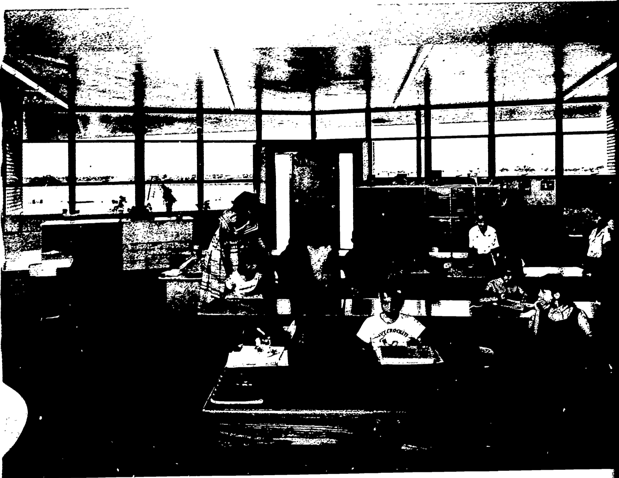
The window wall of a typical Belaire classroom is shaded by the extended overhangs of the roof.
