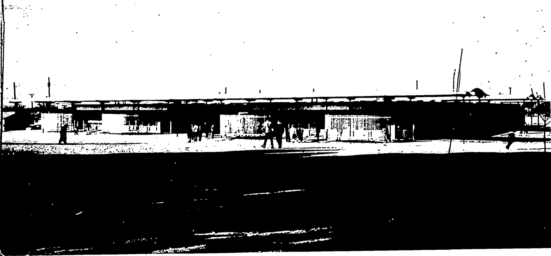
The new Montrose School is an introduction to a different set of standards in Laredo school housing.
