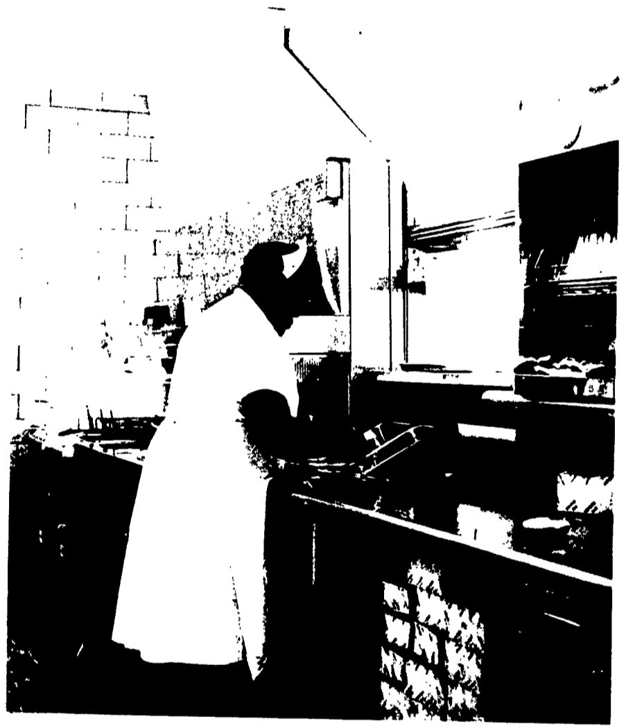
"Spotlighting" a work area to provide the required 20 foot-candles. Fluorescent lighting is considered especially good.
