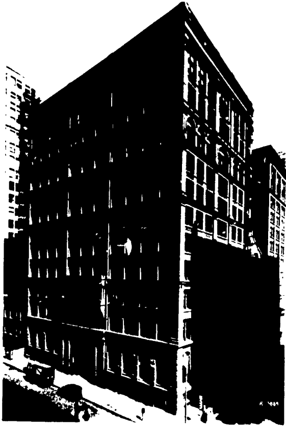
First of the skeletal skyscrapers was William LeBaron Jenney's Home Insurance Building, Chicago, 1885. It was supported entirely by its iron frame.
