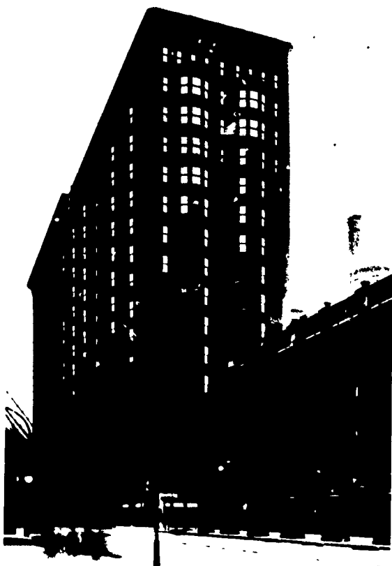
Monadnock Building, Chicago, the last of the great masonry skyscrapers, 1891. Note the thickness of the supporting walls at the ground floor level. Burnham and Root, architects.
