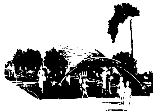
The geodesic dome school built of repetitive mass produced elements, was designed for Kaiser Aluminum Company by Mason, Muntz and Associates, architects.
