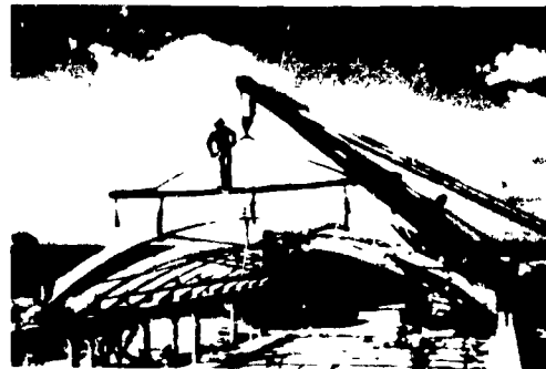
Repetitive elements can save money and construction time by eliminating the custom fitting of each joint.
