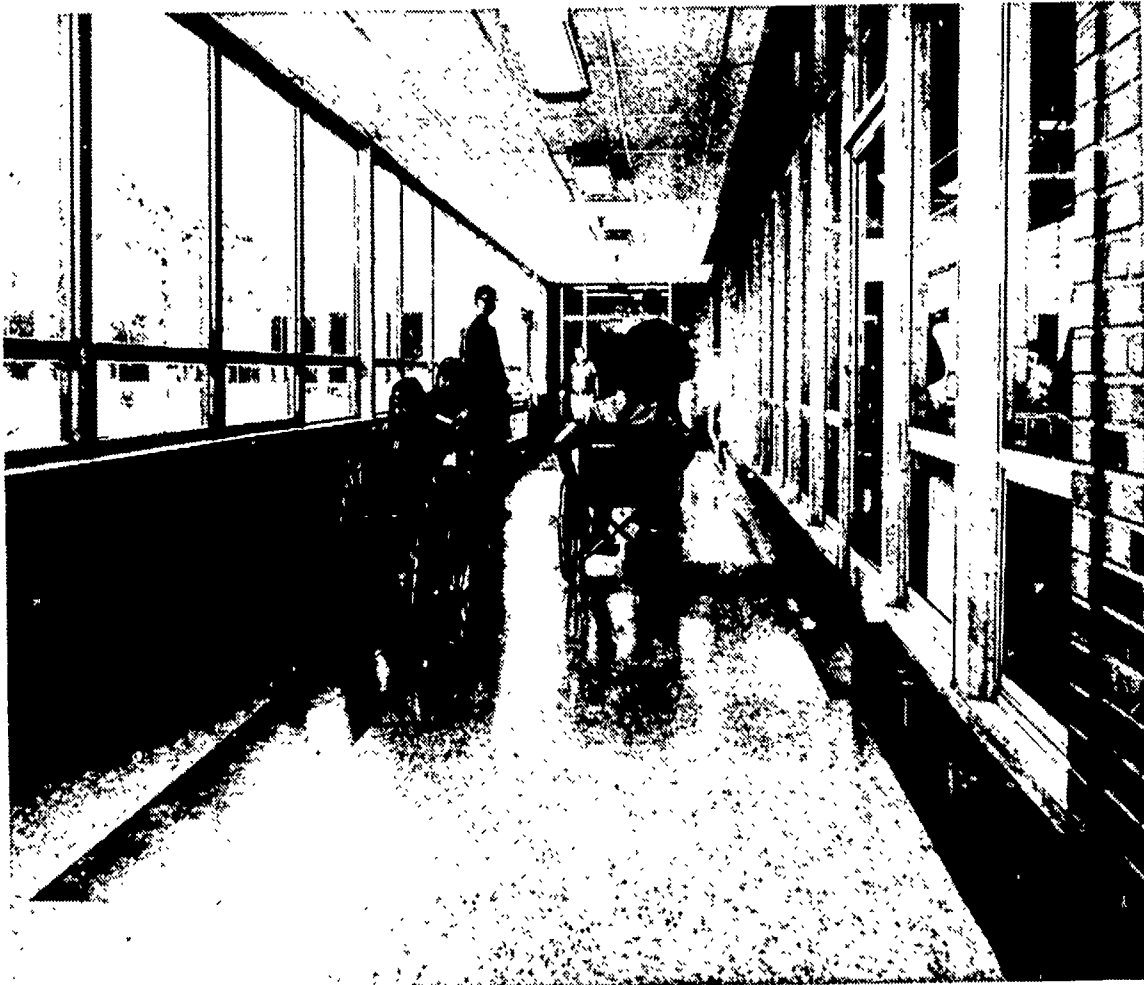
Fig. 3. Major corridors and hallways should be wide enough to allow for two-way wheelchair traffic. The floor should be covered with a non-slip surface material.
