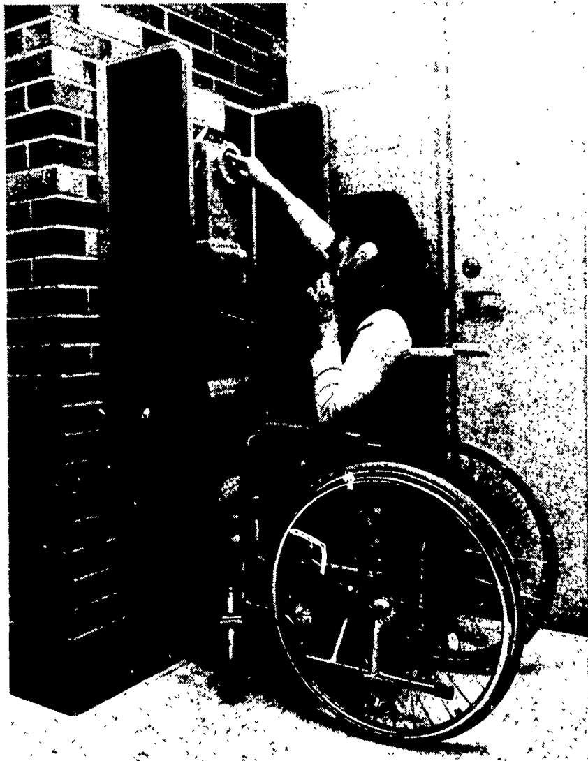
Fig. 1. A lowered public telephone booth for use by the disabled should be located in the building.
