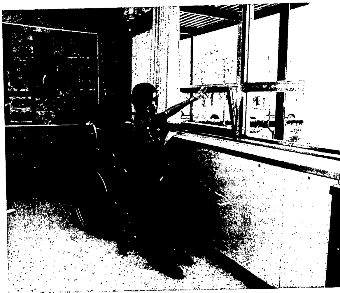
Fig. 5. Classroom windows should be placed at appropriate height for wheelchair students. Cabinets for storage space may be provided below the window.
