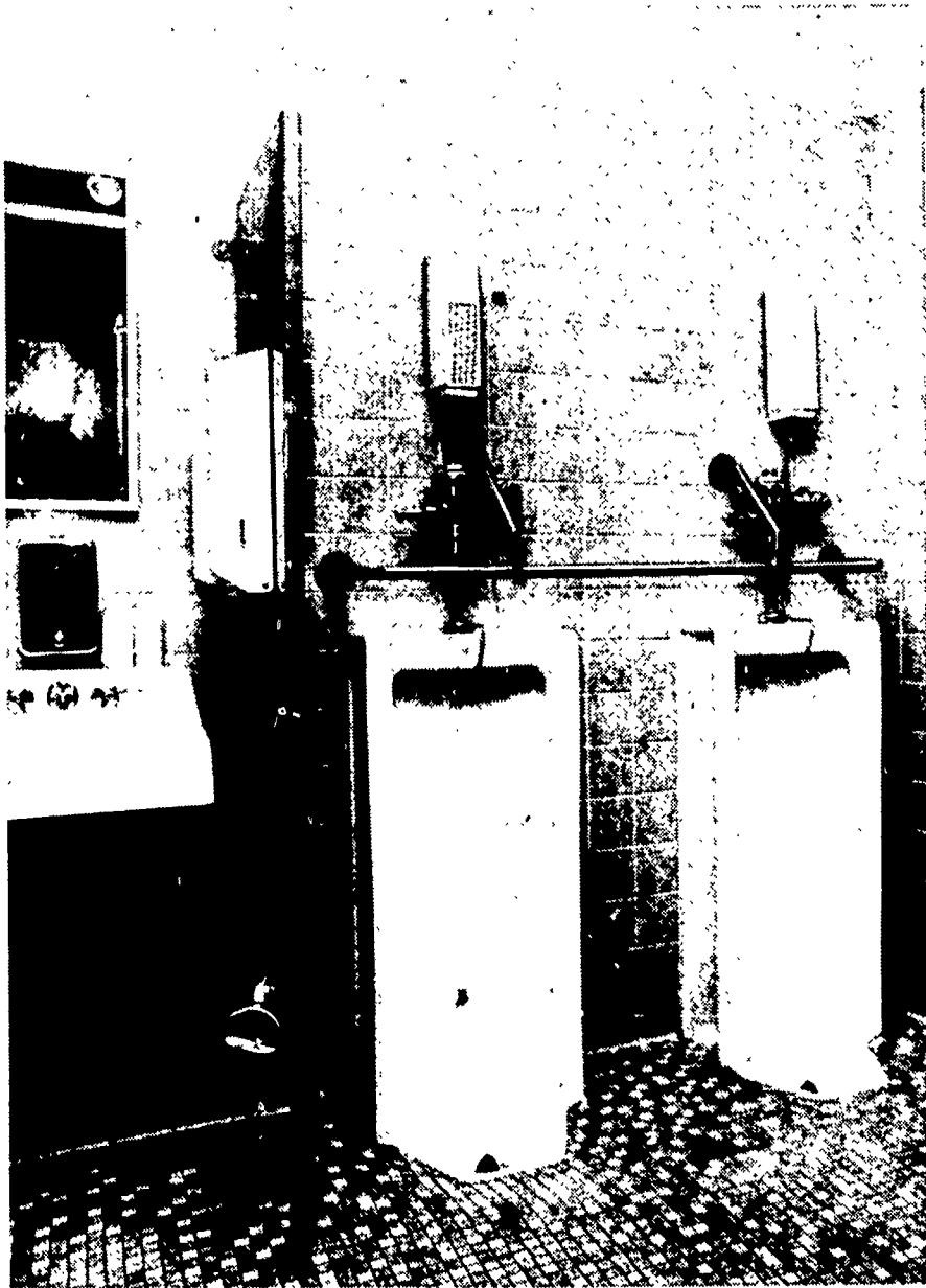
Fig. 10. Wall or floor mounted urinals should be accessible to the physically disabled. Grab bars should be mounted at suitable heights for the age levels being served. Note the male urinal also available for use by wheelchair students.
