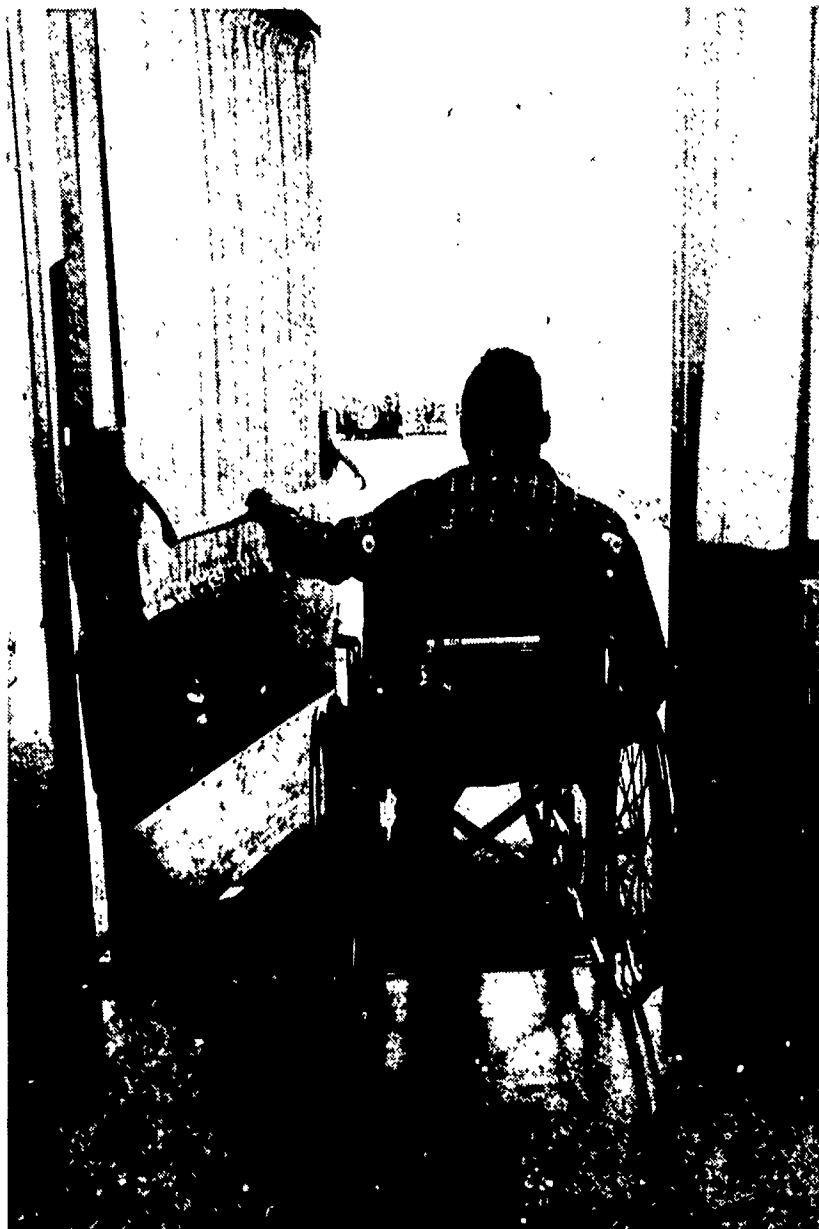
Fig. 4. Exterior doors should be equipped with panic bars for easy opening by a person in a wheelchair.
