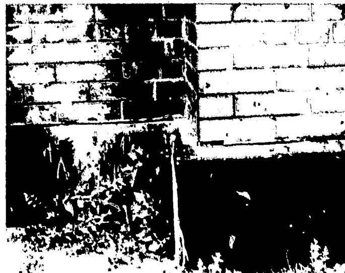
Fig. 2 - Expansion at one end of a 300-foot wall
