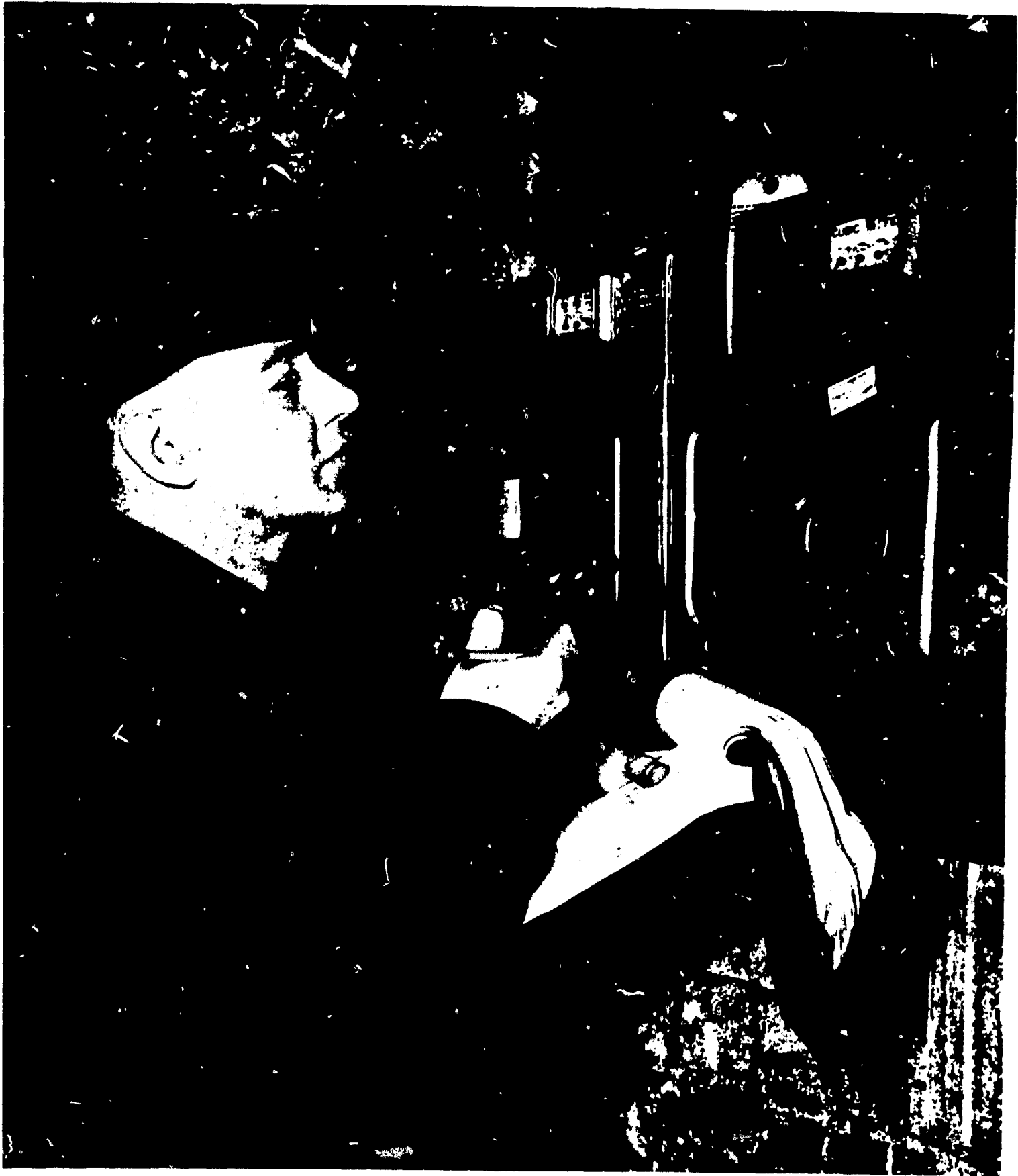
Meter Man Reading a Meter (Consolidated Edison)
