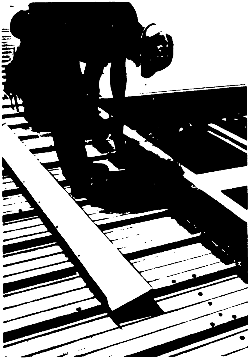
ROOF & FACIA —Precision-fabricated, insulated metal roof systems or built-up roofs of high performance characteristics are available with Space Grid, along with deep fascia panels or two-tone fascia trim.
