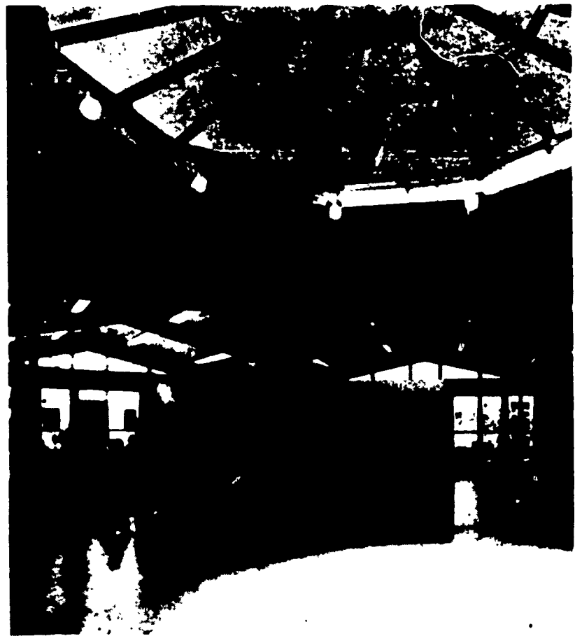
Wood decking, on laminated wood beams, serves as roof and exposed ceiling in central building and wings of Stamford school (photo opposite page). Classrooms open into skylighted multi-use area.
