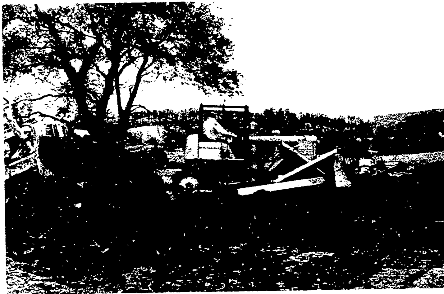
Figure 12. After establishing the desired contour, the topsoil is returned to form the final grade.
