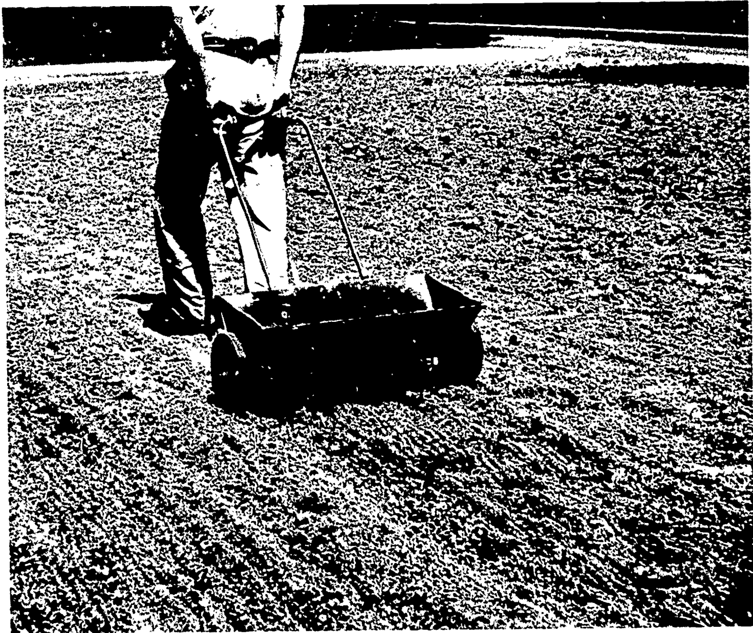
Figure 20. Starter fertilizer is spread over the seedbed prior to finish grading.
