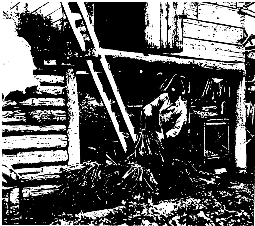
Storage sheds in native villages are built on stilts as a protection from marauding animals. The man is preparing to store a supply of dried fish for feeding sled dogs in winter. PHOTO: DEPARTMENT OF THE INTERIOR
