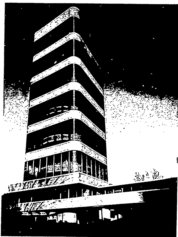
Figure 1-- Over 133,000 feet of glass tubing in this 154 foot tower require sealing.
