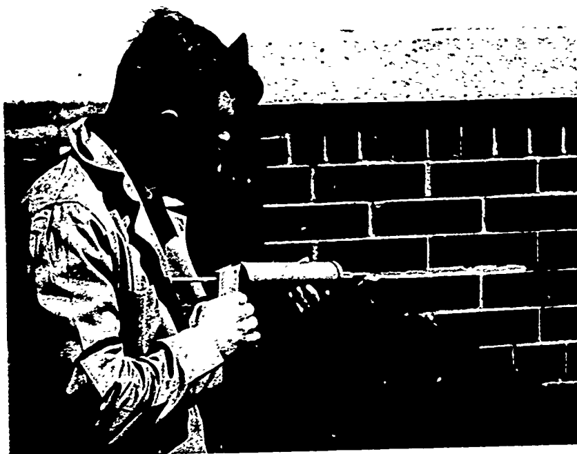
Figure 5 -- Application of non-sagging epoxy sealant.
