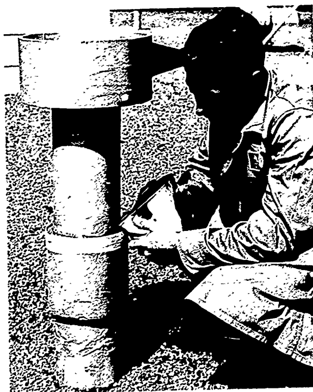
Figure 6 -- Application of self-leveling epoxy sealant to pipe joint.
