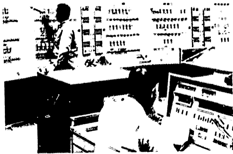
Operators oversee computer console which monitors chemical plant conditions and types out operating log sheets.
