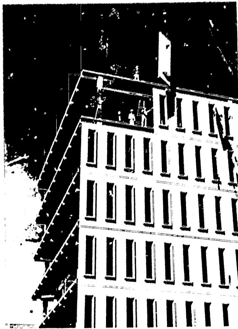
Precast concrete structural wall panels are lowered into place.
