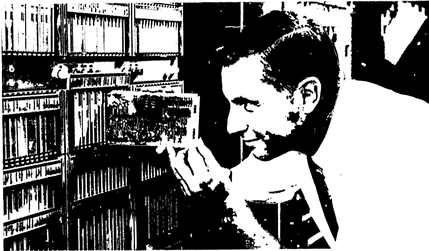
Defective circuit card is replaced in telephone electronics central office after being located by computer.
