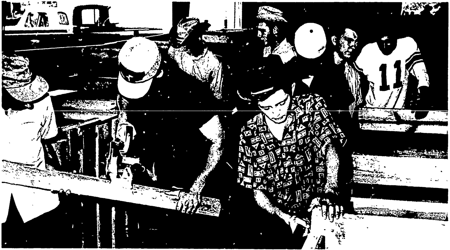
NYC enrollees in Tishomingo County, working on a county fair building. Without the assistance of the NYC enrollees the building would not have been ready for the fair.
