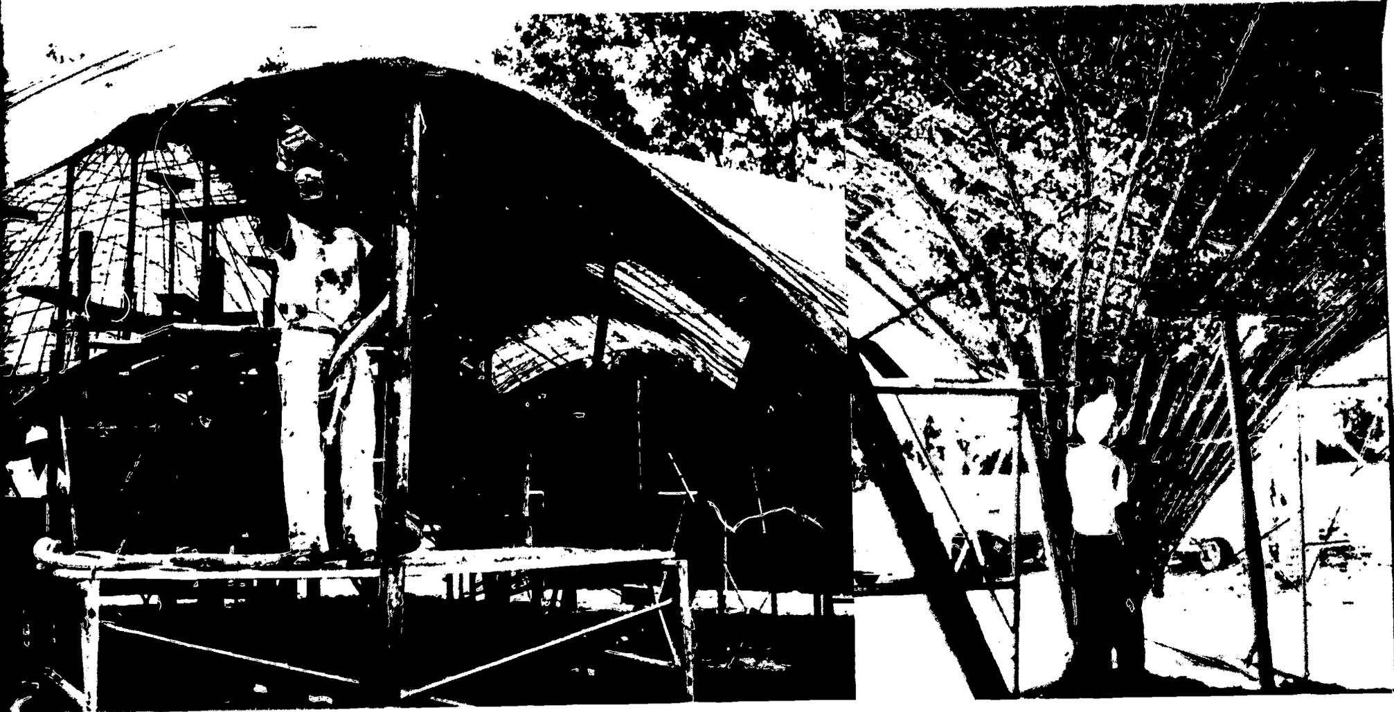
The first coat of concrete was rather thin and intended primarily to fill the voids in the metal lath, thus providing a backing for the application of succeeding coats of concrete. The plasterers worked from day to day spraying onto the underside of the armature in a continuous rotating pattern. Not until the underside concrete work was complete, except for the finish coat, did the plasterers take their equipment to the top side of the armature.
