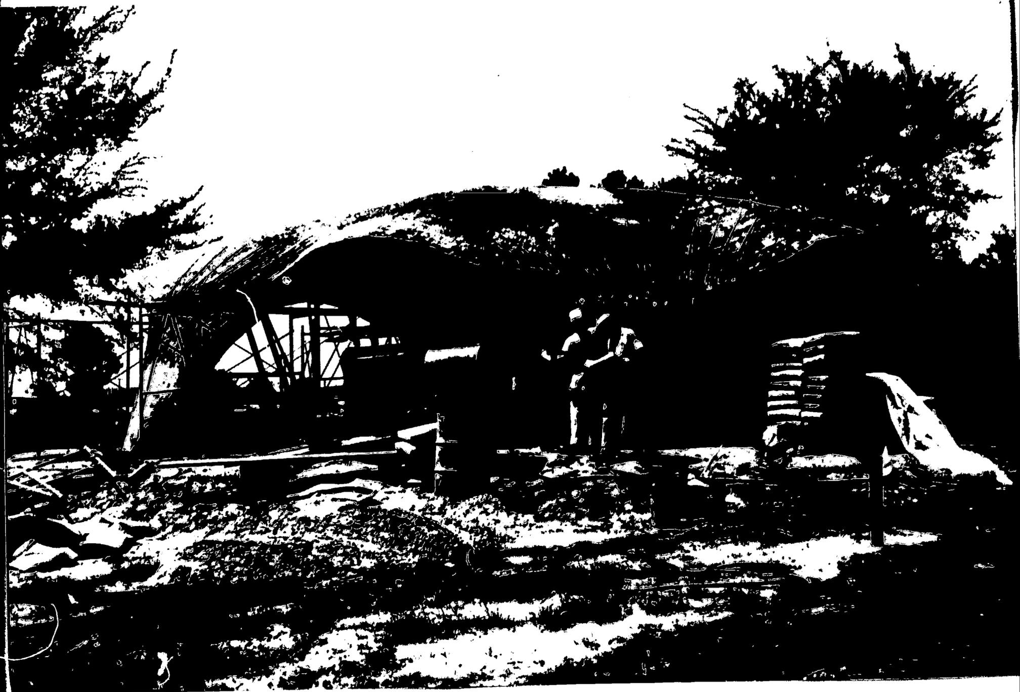
To get the concrete mix to the top of the dome it was pumped there using the spray machine without the hose nozzle itself. As the concrete was pumped in a steady stream onto the surface by one man, another man spread the mixture around with a long straight float. As the mixture began to harden it was sculptured to its finished shape by the plasterer and his apprentice using hand tools.
