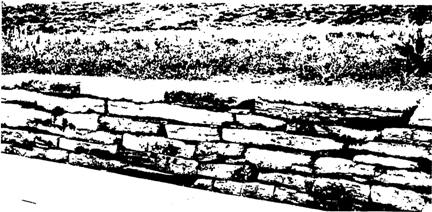
Figure 41. A dry wall is attractive, inexpensive, and easily constructed.
