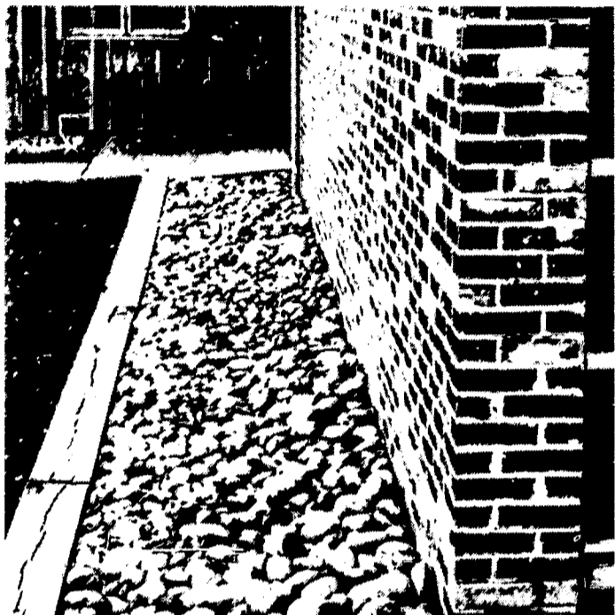
Figure 49. Loose stones fill a space kept dry by the roof overhang.
