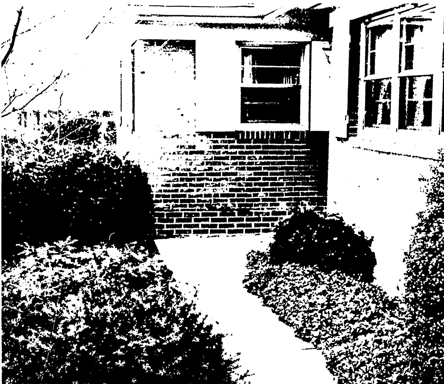
Figure 21. An attractive entrance planting.
