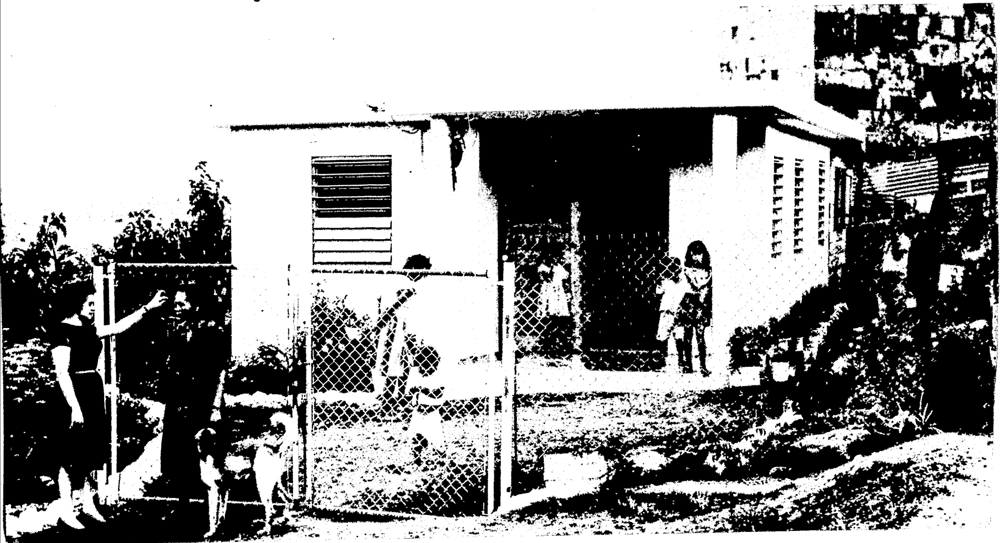
Figure 21—One of the new houses built with the help of the Social Program's Administration.
