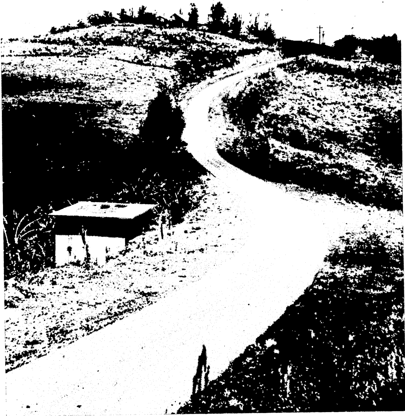
Figure 20—View of the same road, now paved.
