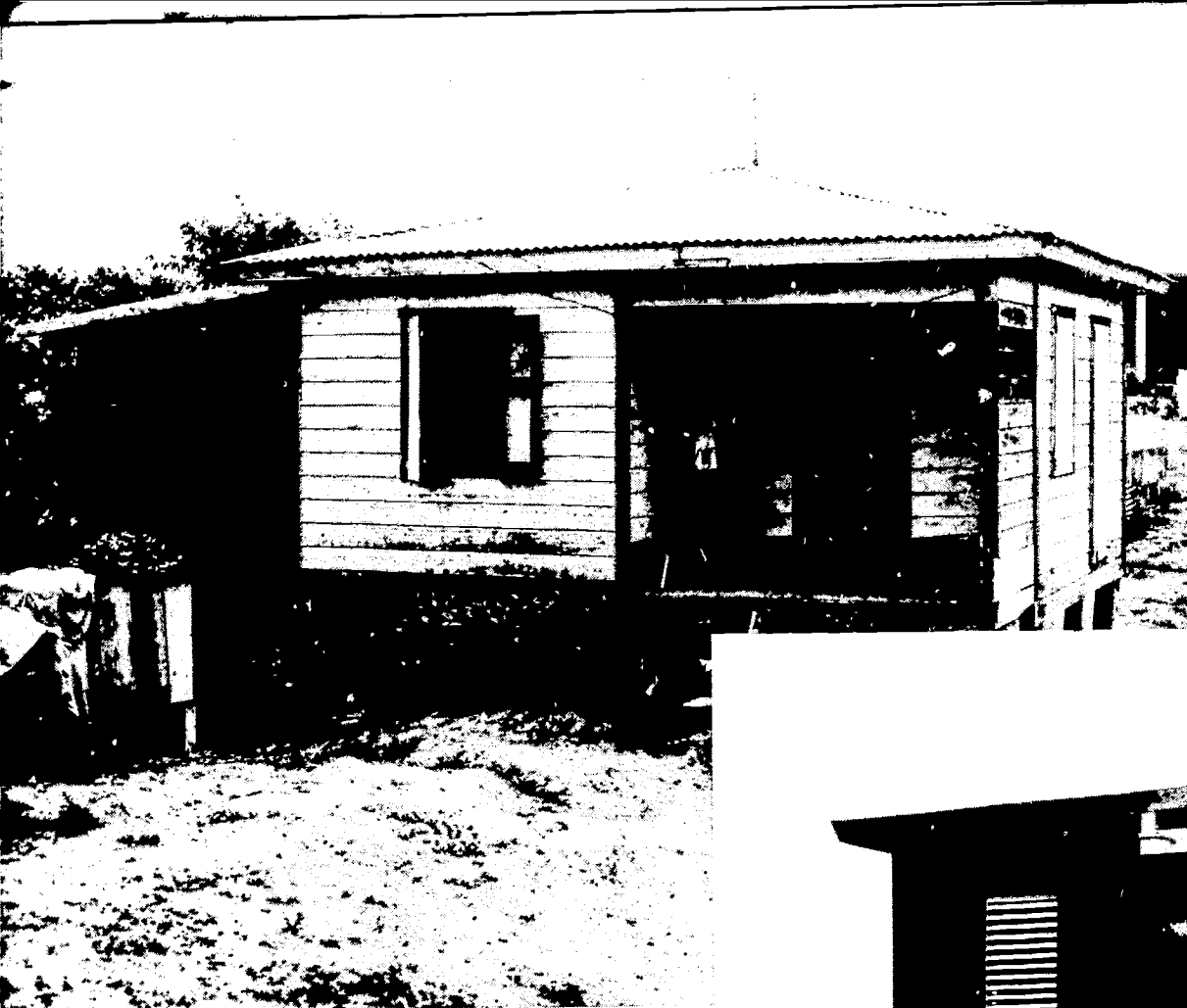
Figure 22A—The old house.
