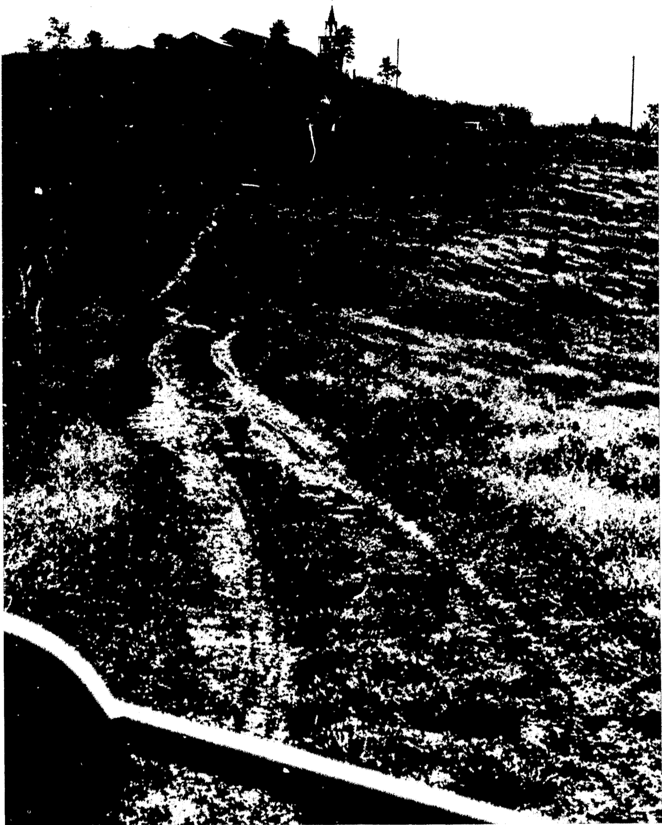
Figure 19—A sample of the old rutted, muddy road.
