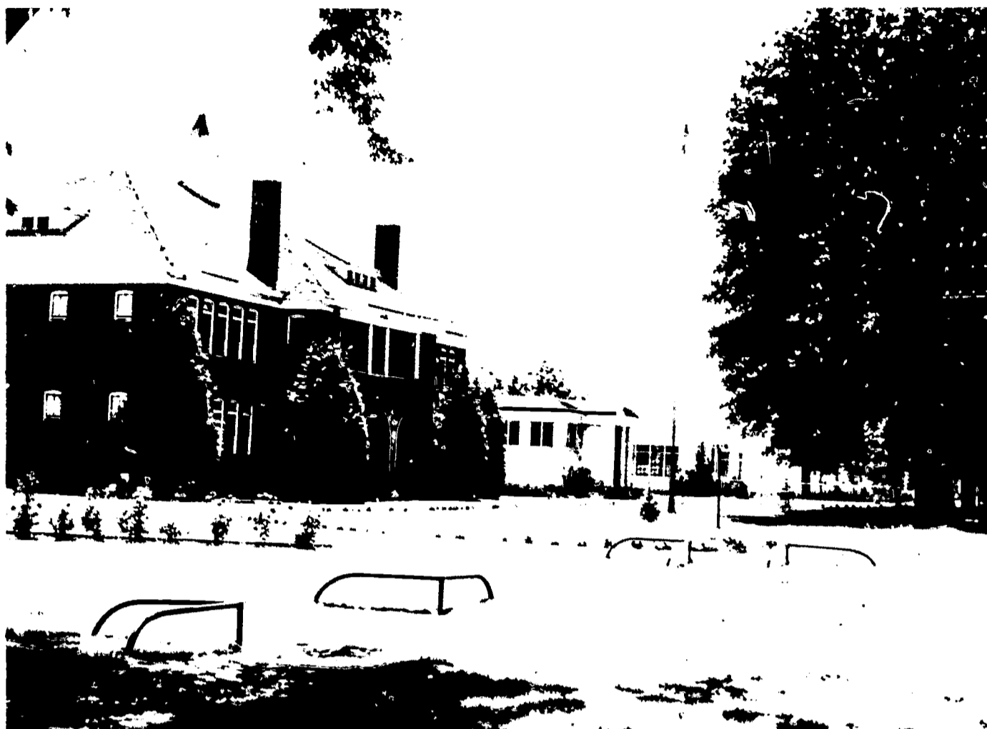
Special Navajo Program classroom buildings at Chemawa Indian School
