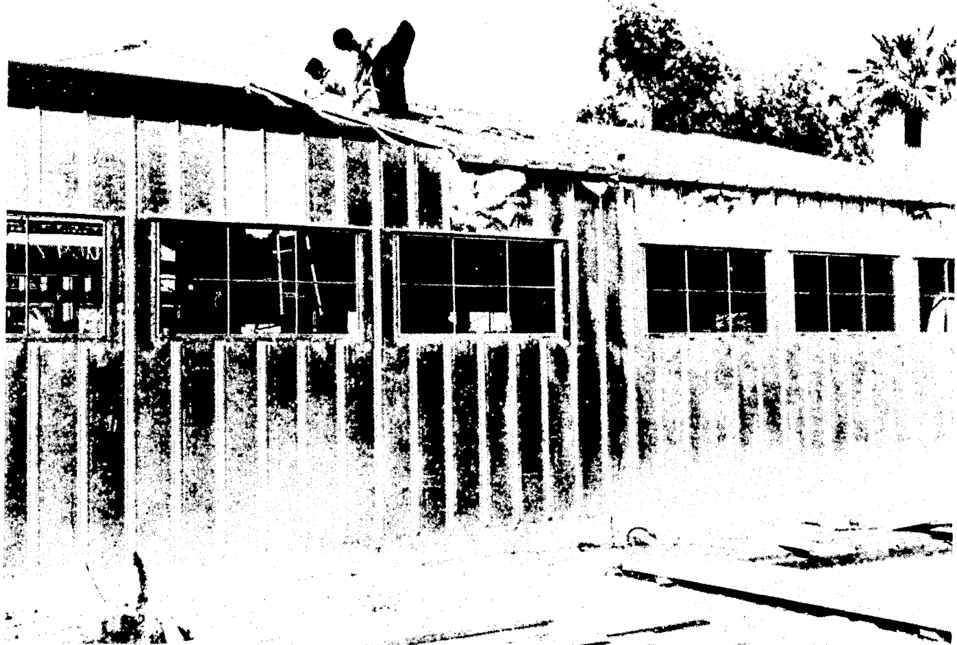
Sheet metal work
