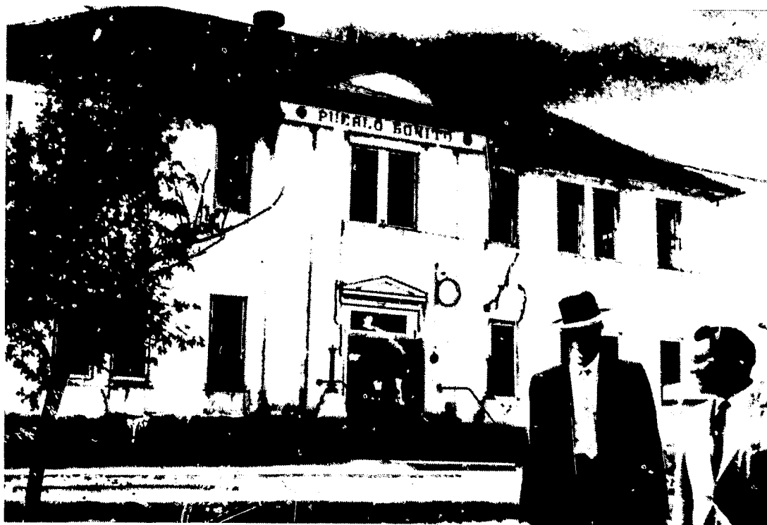
The old Crownpoint (formerly called Pueblo Bonito) Boarding School ended its 52-year career in Navajo education at the close of the 1960-61 school year. A new, modern school plant will replace this antiquated and unsafe structure.
