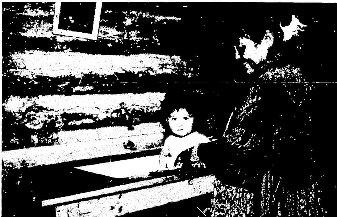
(Upper) Inside the hogan, a water faucet provides a protected water supply for various domestic uses. The sink units with subsurface waste disposal, is part of the project.
