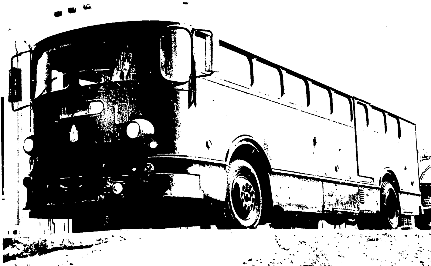
NMSU Mobile Instructional Facility, Before renovation
