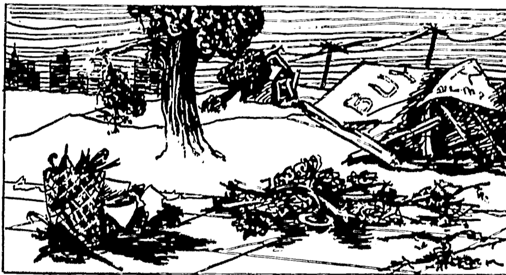
After the hurricane.
