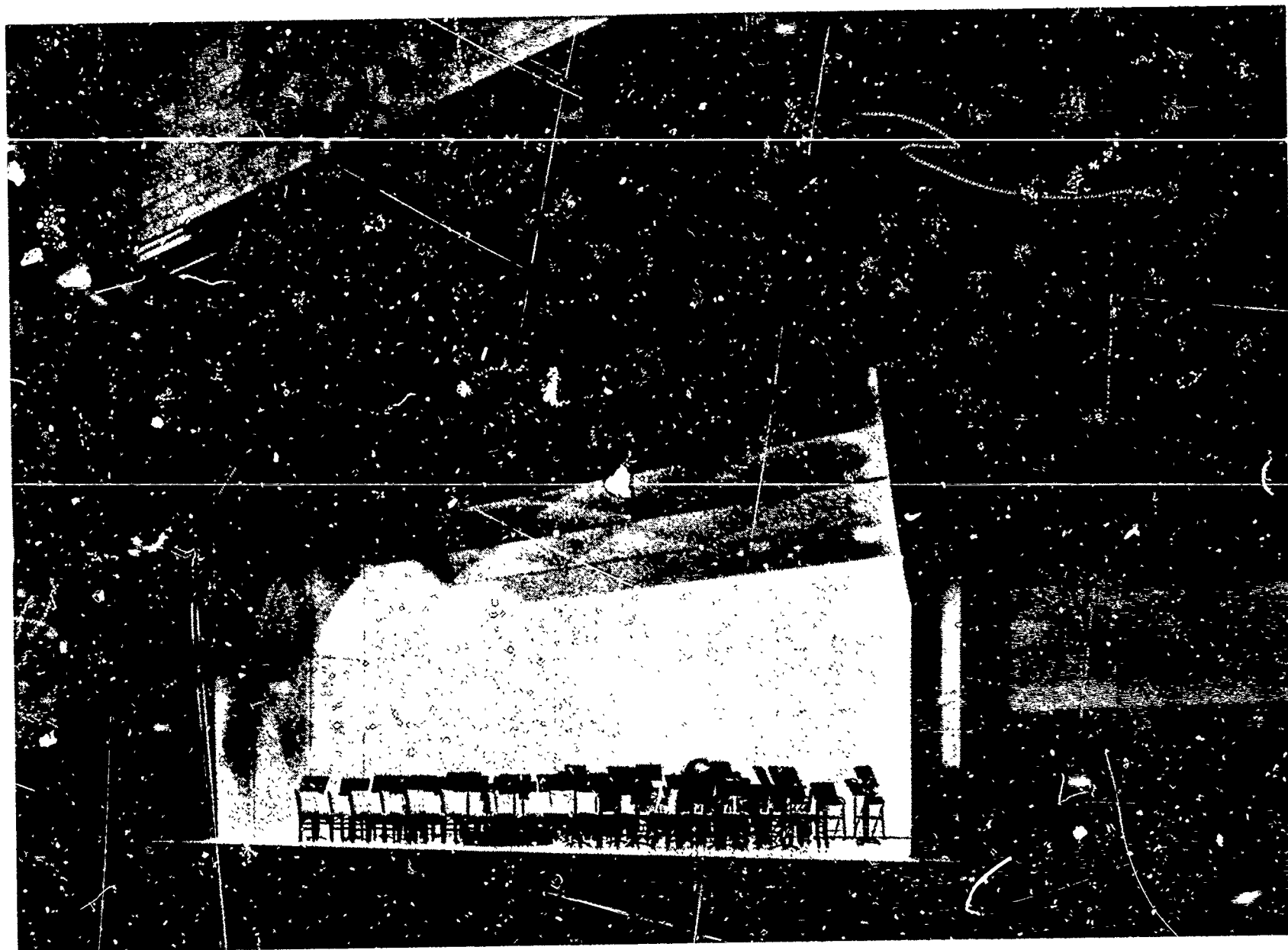
The orchestra enclosure in a stagehouse should be fairly tight with a minimum of openings to the backstage area. Michigan State University Shell by Stagecraft Corporation
