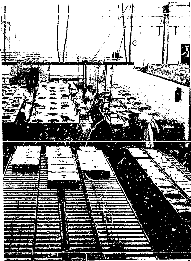
THE LOADING AREA. CARTS ARE HEATED FROM OVERHEAD ELECTRIC CABLES AND CHILLED BY DOLE PLATES.
