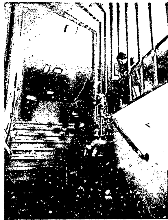
short stair runs, rails both sides
