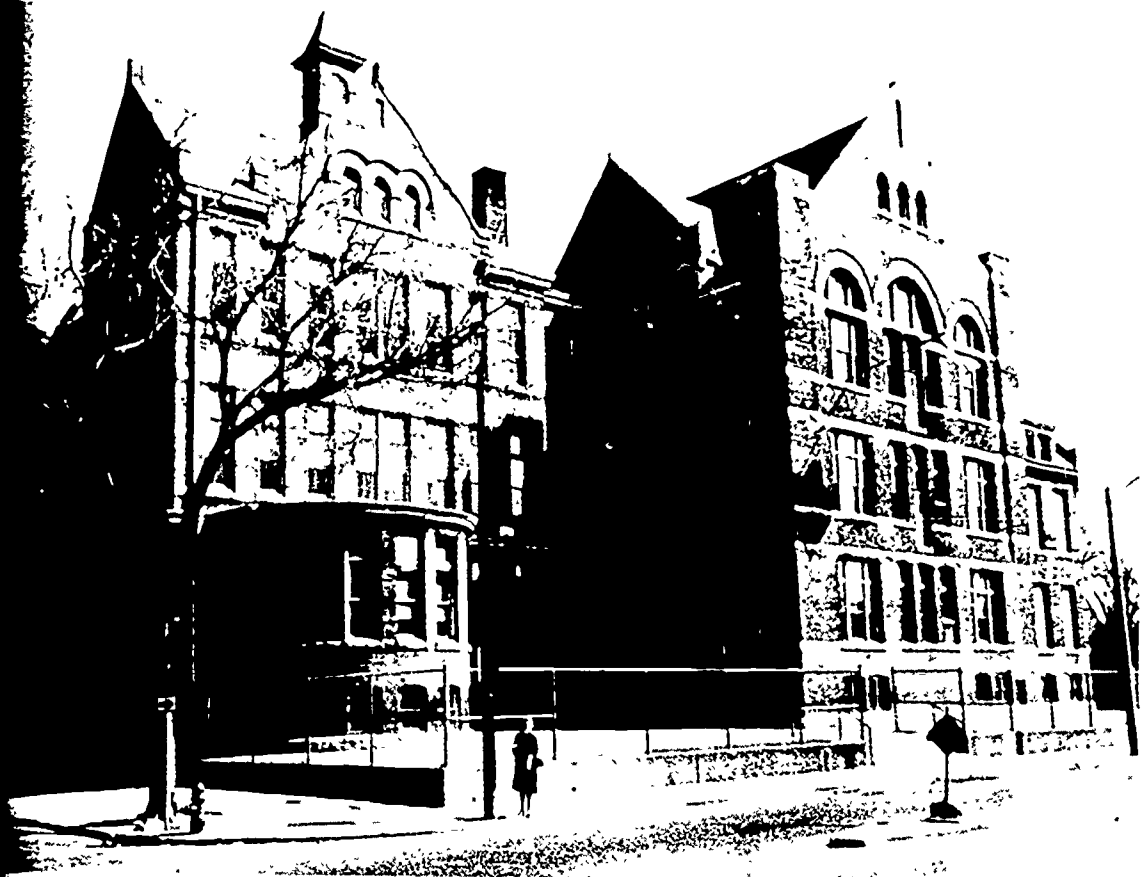
Typical older school in Milwaukee -- this one built in 1887. The city now has a budget of approximately $1,500,000 annually to add years of life to schools like this.
