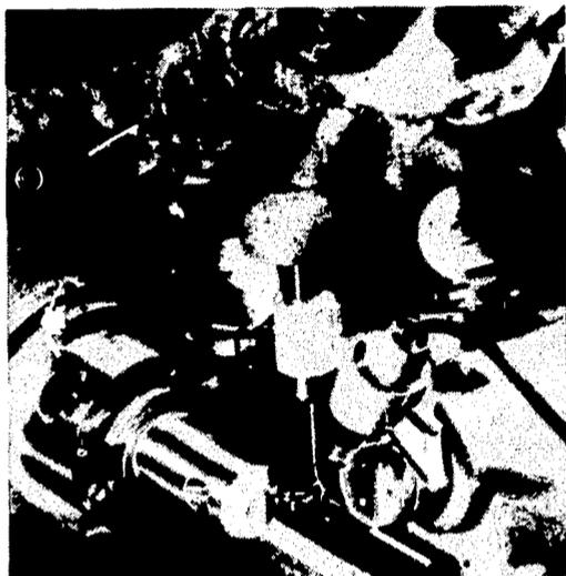
Fig. 4—10. Verifying boring tool offset with optical viewer
