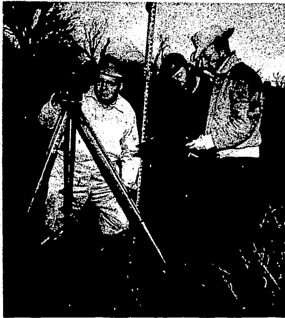
Soil Conservation Service engineers prepare to stake out a pond according to the landowner's conservation plan.
