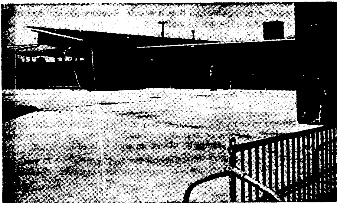
NEW SCHOOL BUILDING WITH PAVED PLAY AREA
