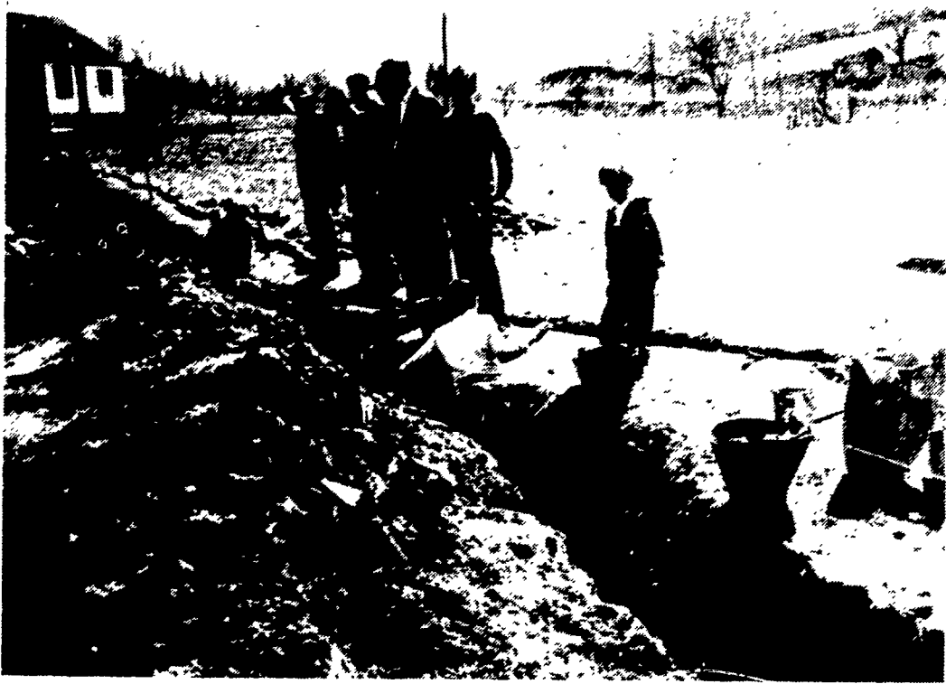
Pupils and parents work cooperatively to provide playground drainage.
