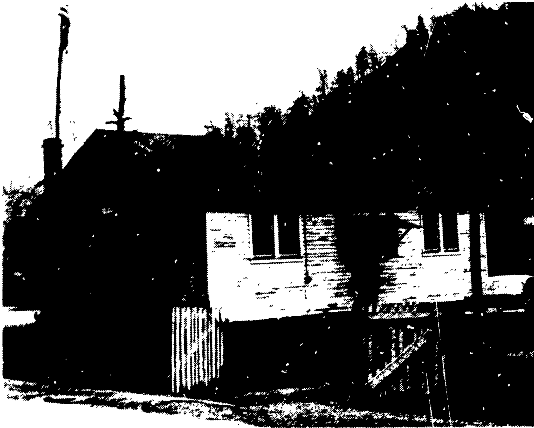
Unimproved building and grounds early in RSIP.
