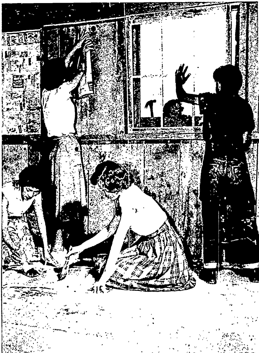
Repairing a farm worker's cabin.
